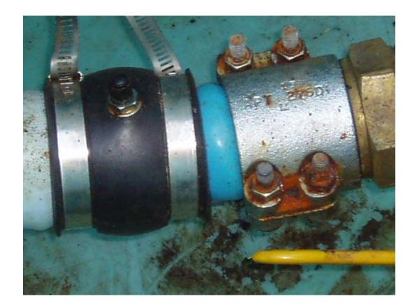
Piping interstitial space is open to the sump (Open systems only, N/A if closed system or not conducting interstitial monitoring)
