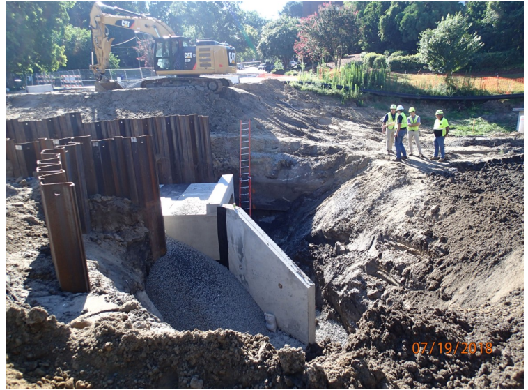
The City of Greenville constructs the Town Creek Culvert project (CS370487-10)
