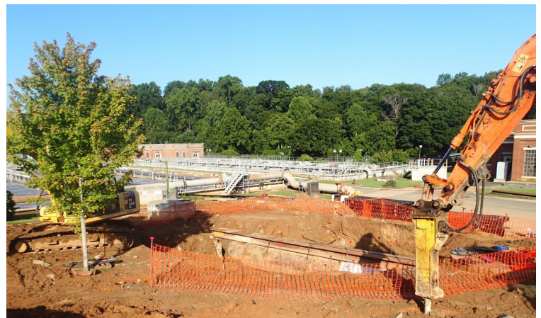
Construction at the Sugar Creek WWTP in Charlotte, NC (CS370377-14)
