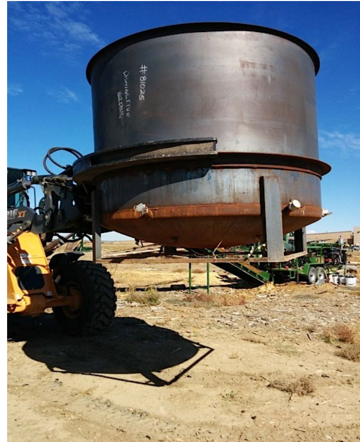
Loader Transporting Kiln to the Enclosed Product Handling and Packaging Area
