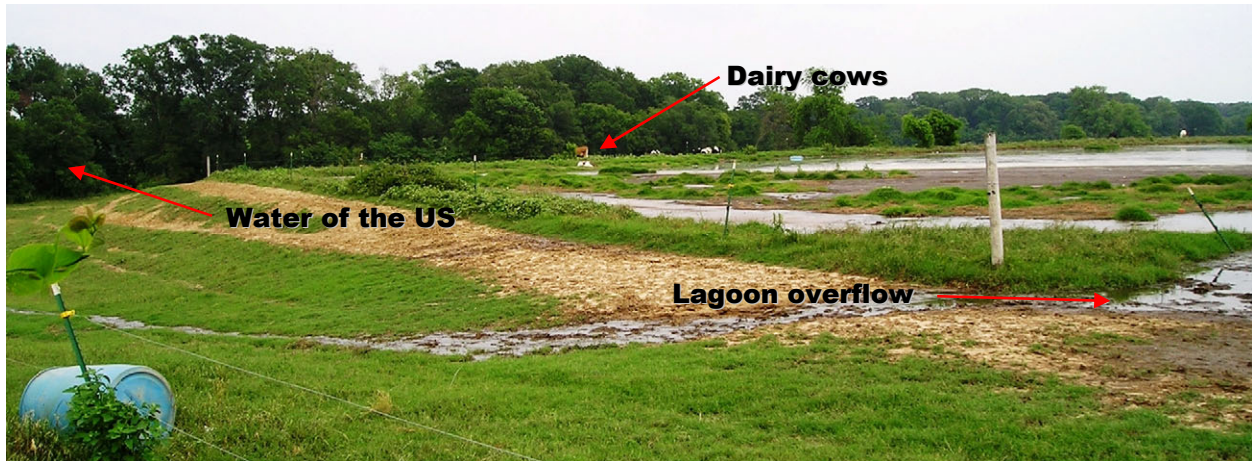
Photo 2. This lagoon at a dairy CAFO is upslope from a water of the U.S. and overflowing. In addition, cows stand on the embankments of the far side of the lagoon, which may degrade the embankments over time, and vegetation is growing in the lagoon, which indicates poor maintenance. (Source: EPA Region 6.)
