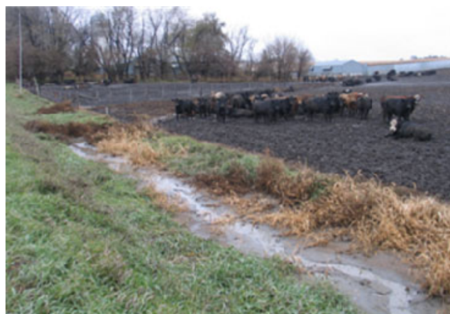
Photo 7. This section of the beef feedlot production area has an outlet for manure and process wastewater to a roadside ditch. If the ditch is, or conveys process wastewater to, a water of the U.S., then the CAFO discharges or proposes to discharge. (Source: EPA Region 7.)
