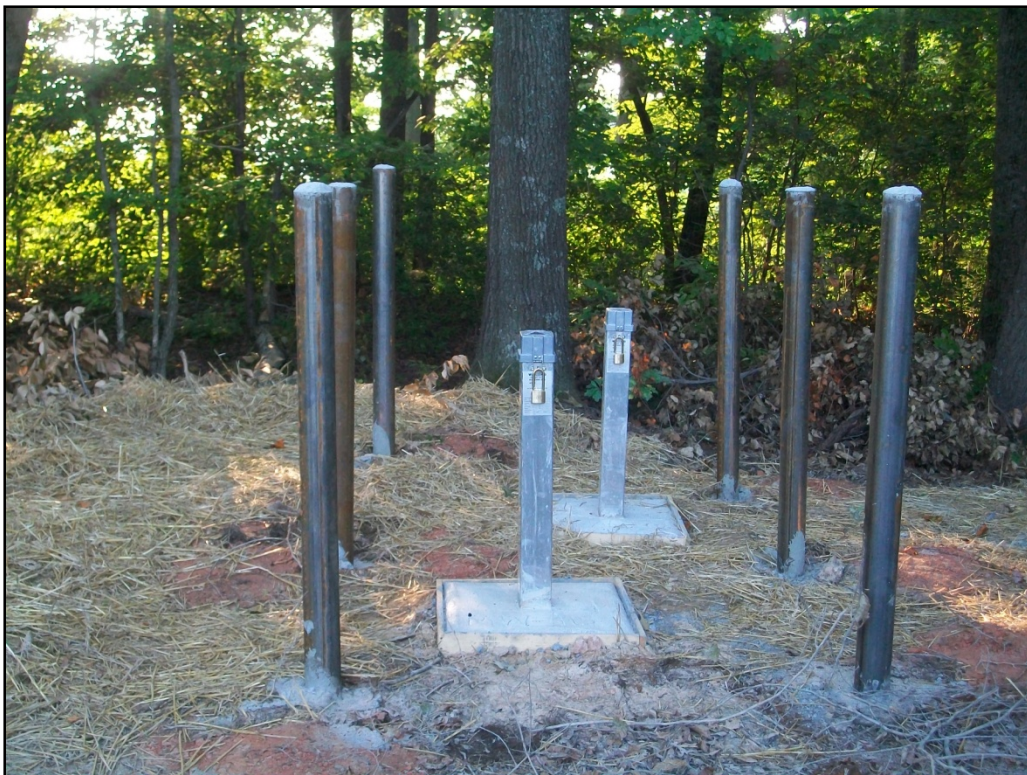
Photo 4: Well pair MW-11S (Left) and MW-11D (Right)
