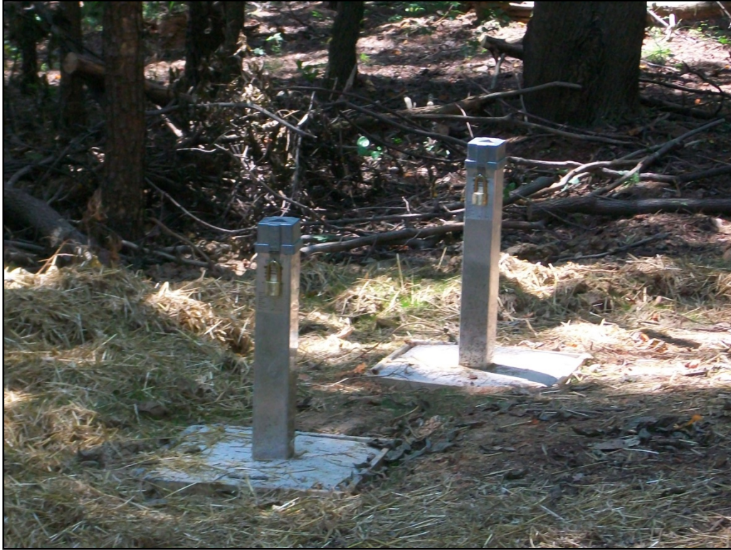
Photo 5: Well pair MW-10S (Right) and MW-10D (Left)
