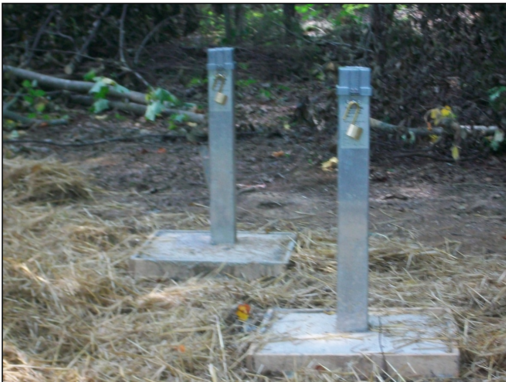
Photo 2: Well pair MW-12S (Right) and MW-12D (Left)
