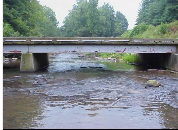
Buffalo Creek at SR 1504, Caldwell County.
