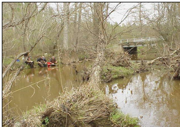
Upstream view (looking downstream) of Hamer Creek at SR 1159, Richmond County.
