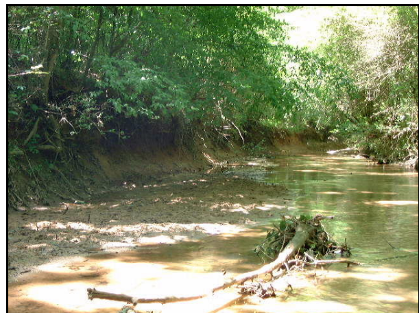
Vertical and eroding banks at Catawba Creek at SR 2435, Gaston County.
