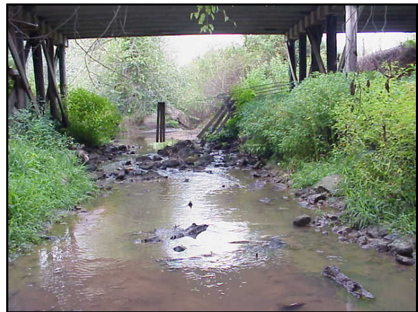
Riffle at bridge in Muddy Fork at SR 1438, Alexander County.
