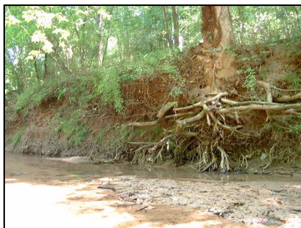
Figure 4. Entrenchment and vertical eroding banks, Catawba Creek, SR 2435, Gaston County.
