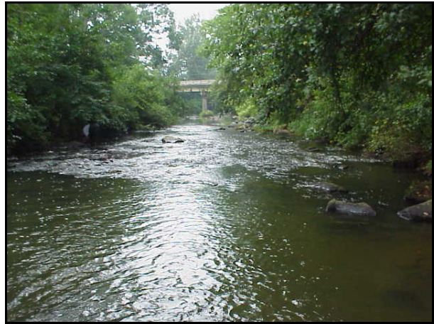
Linville River at US 221, Avery County.
