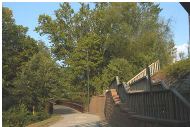
Glenwood Avenue, Raleigh - Phytoremediation
