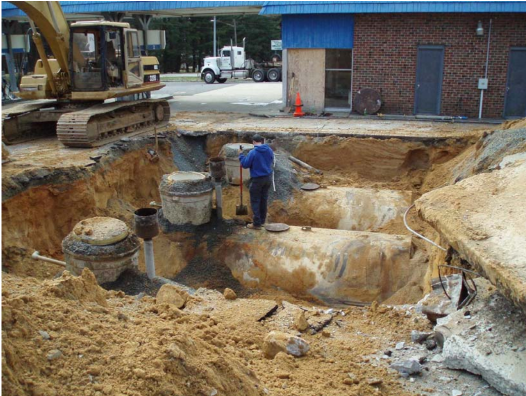
UST Release Incident-Tank Removal
