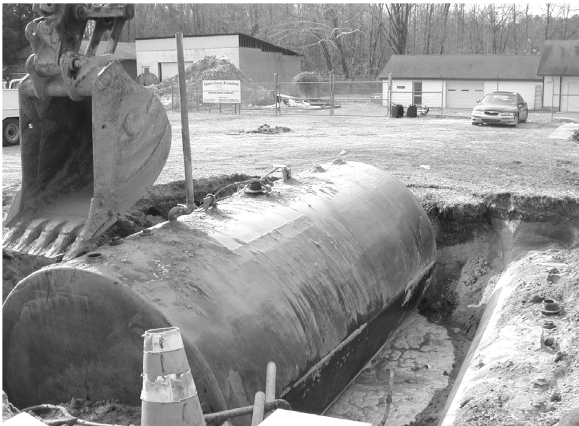
UST Release Incident-Kerosene Free Product in Basin
