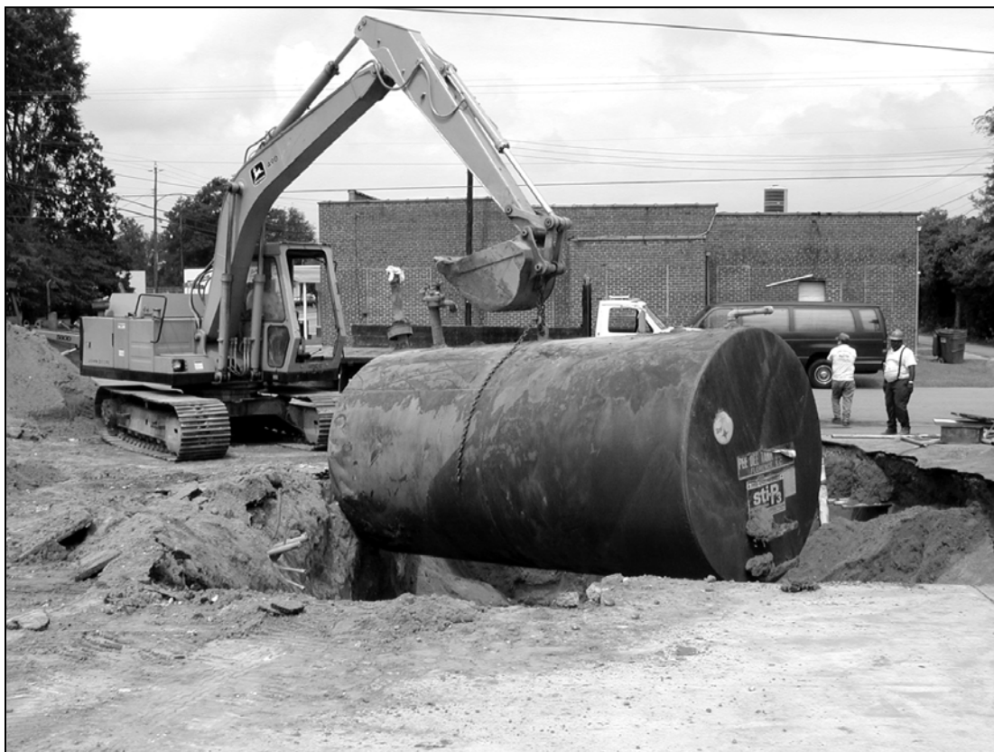
UST Release Incident-Tank Removal
