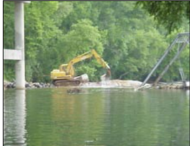
Construction in the Broad River at SR 1106, Rutherford County.
