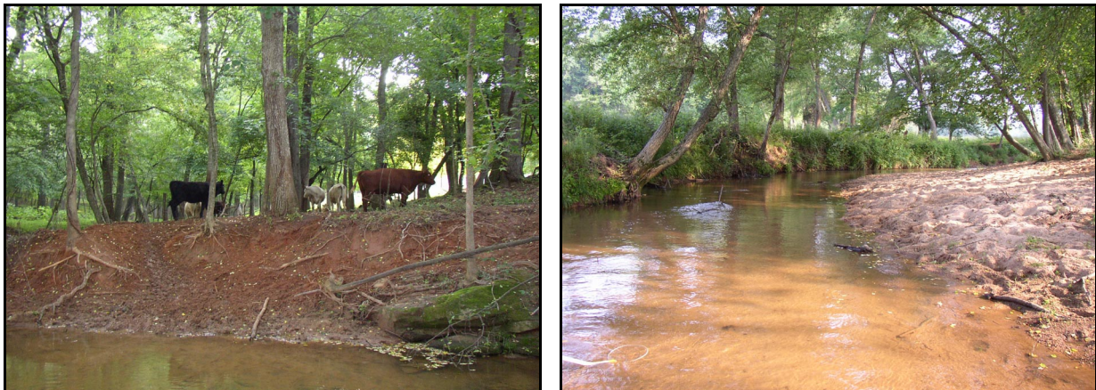
Figure 4. Livestock with access to the stream, sandy substrates with few riffles, and eroding and sloughing banks, Sandy Run Creek at SR 1332, Cleveland County.
