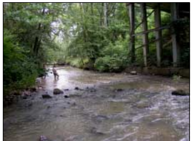
Marys Creek at SR 2174, Alamance County.
