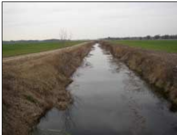
Figure 98. Lyons Swamp Canal, NC 11, Bladen County.
