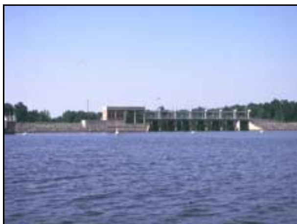
Figure 31. Dam at Cane Creek Reservoir, Orange County.
