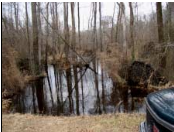
Lillington Creek, SR 1520, Pender County. Upstream of bridge, the channel is less distinct.
