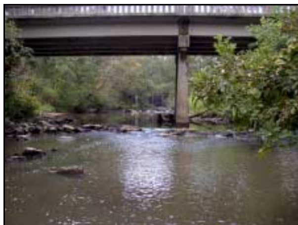
Upstream view of Haw River at NC 87, Alamance County.
