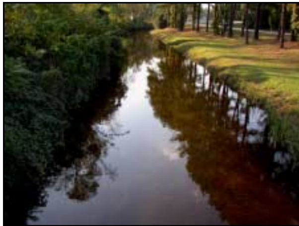
Cross Creek at NC 87/210/24, Cumberland County.
