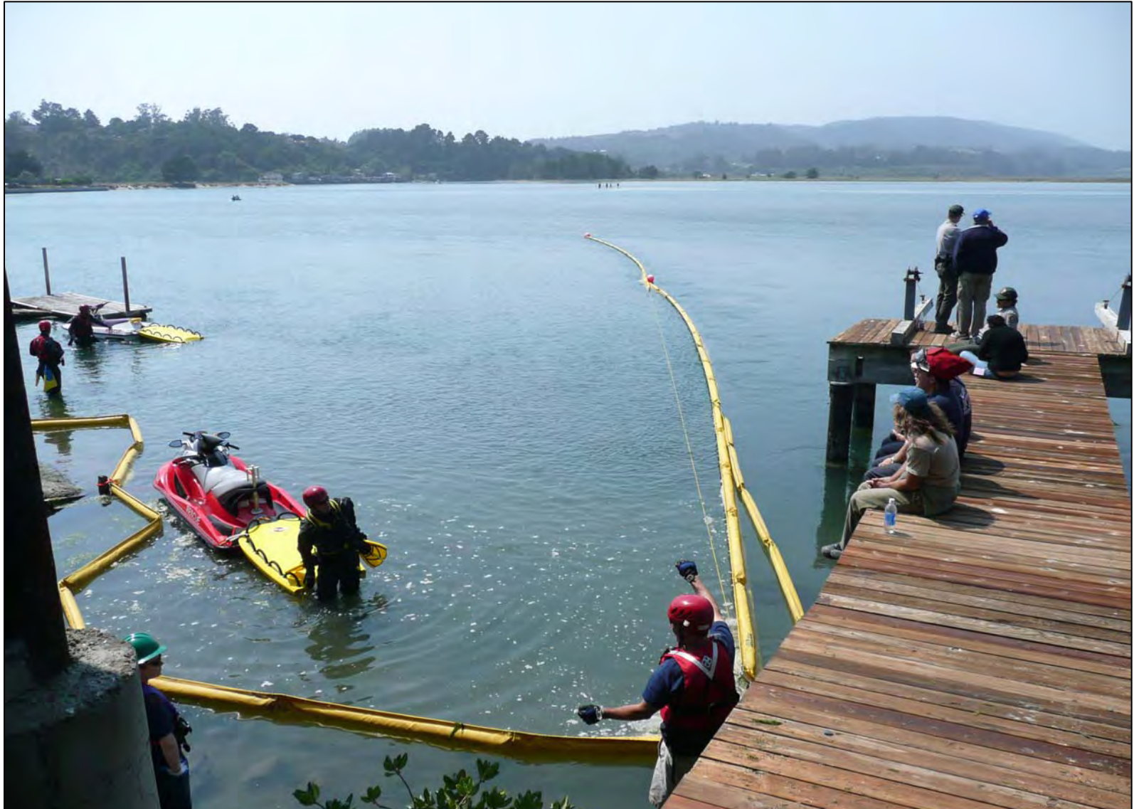
Shoreline Containment & Protection Boom Being Deployed
