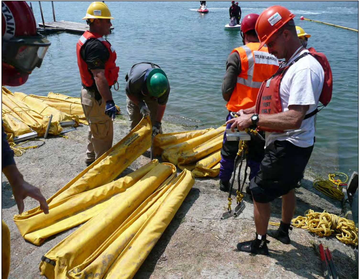
Boom in 100' Lengths is Zig-Zagged on the Boat Ramp in Seadrift
