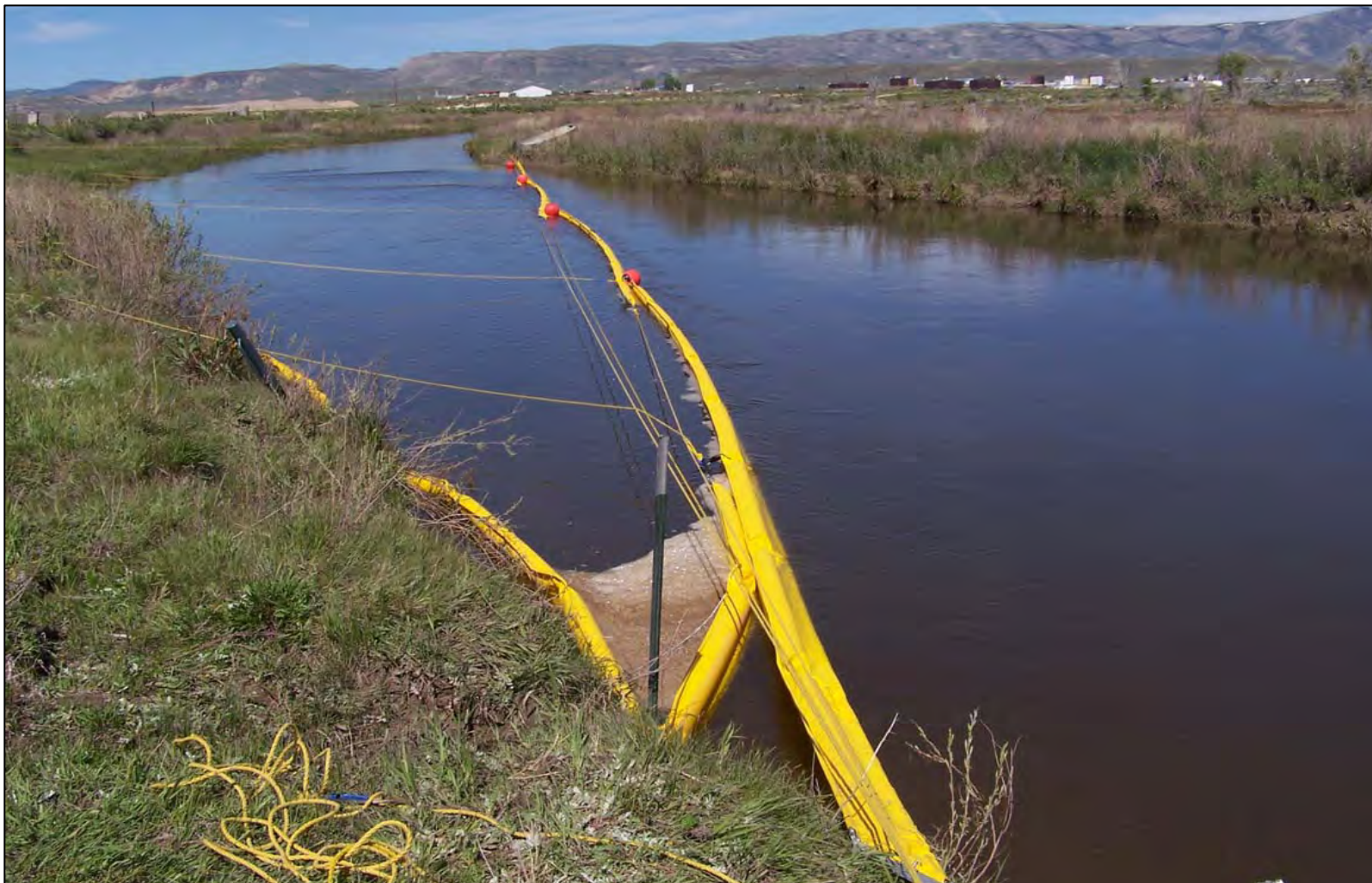
Cascade Diversionary Boom Deployment with Shoreline Protection Green River - La Barge, WY
