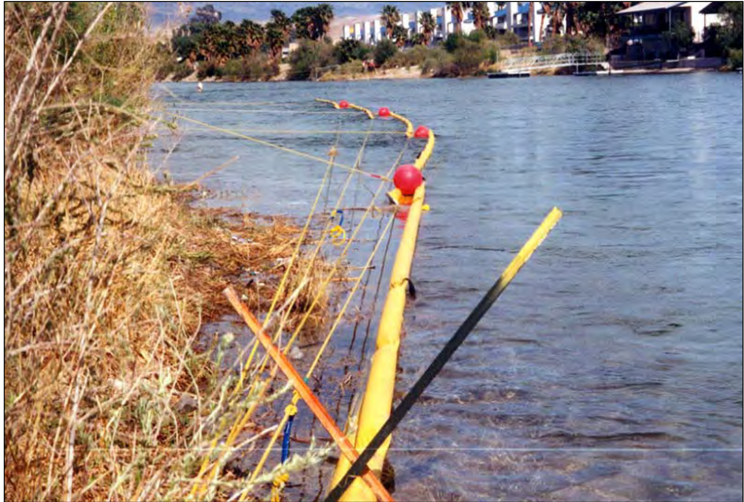
Cascade Diversionary Boom Deployment Colorado River - Laughlin, Nevada
