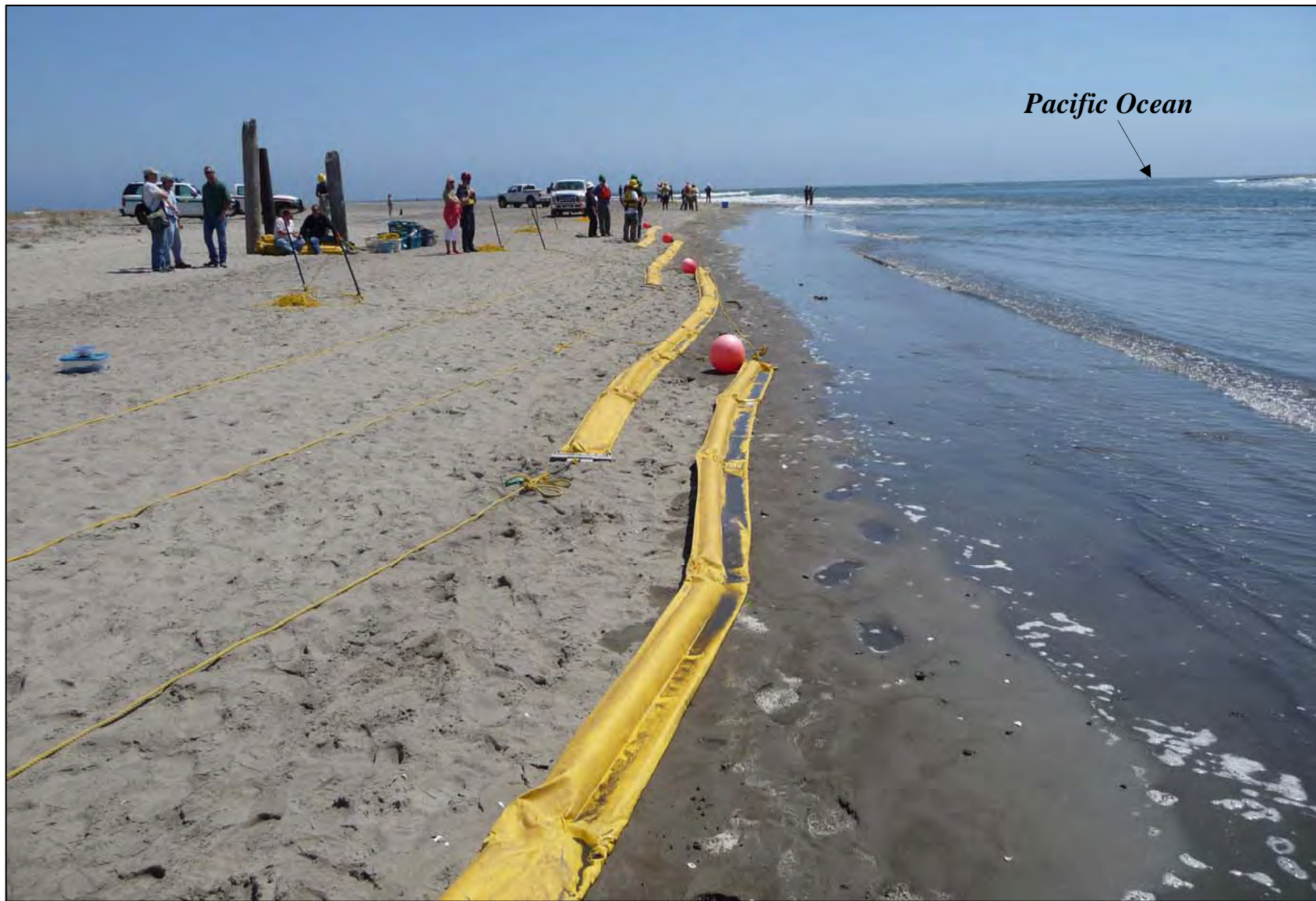
Boom Laid Out Along the Shore Preparing to Deploy Cascade System - 1 st Exercise
