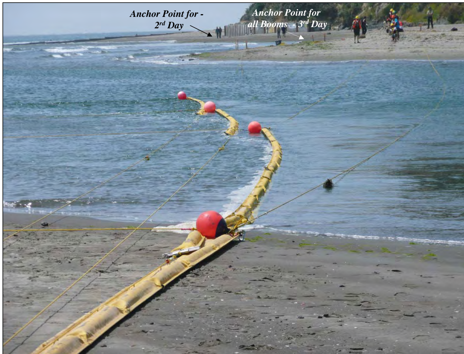
Four Booms Deployed - Containment of Rice Hulls Beginning
