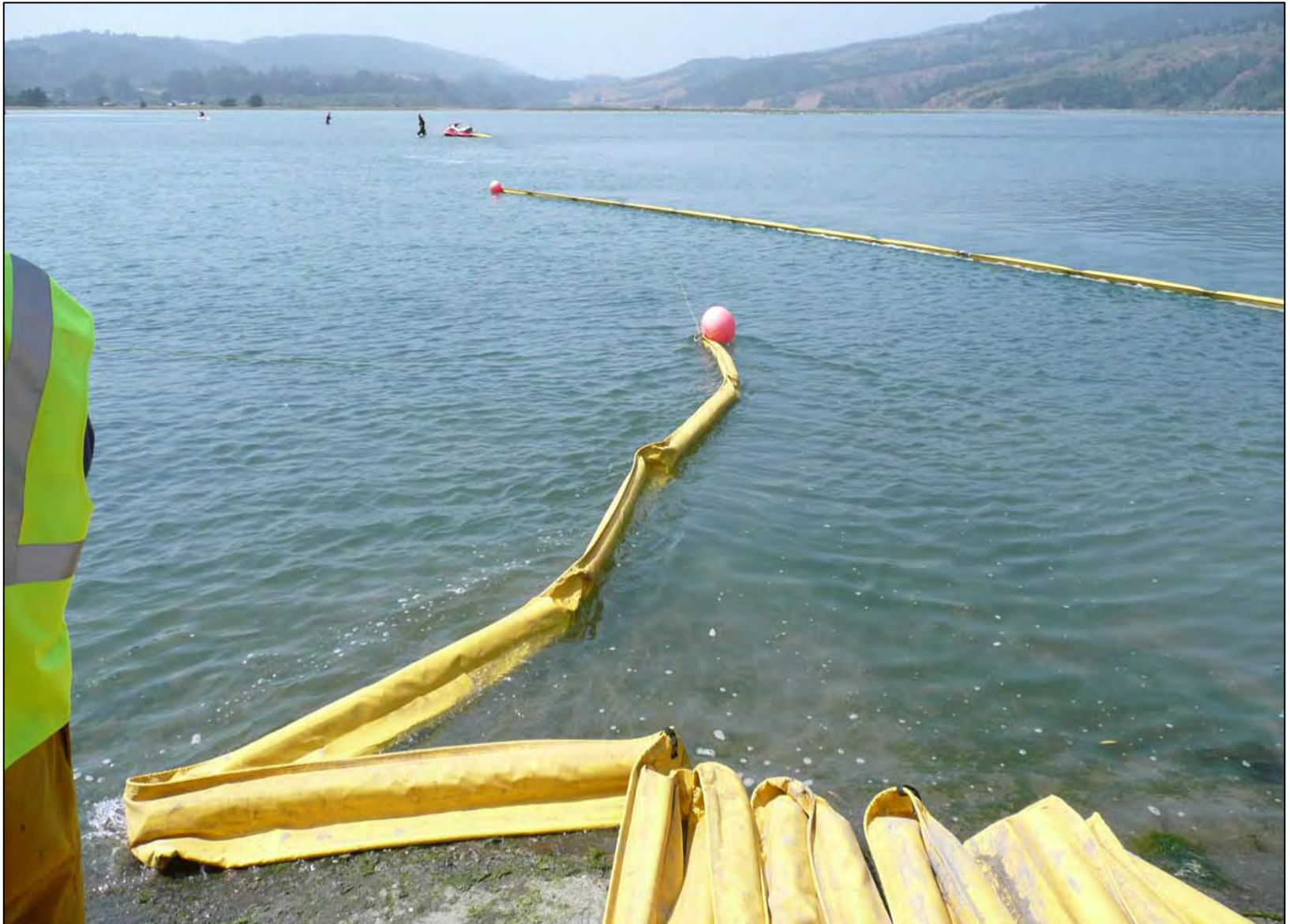
Team on Sandbar Island Pulls Line and Boom is Being Deployed
