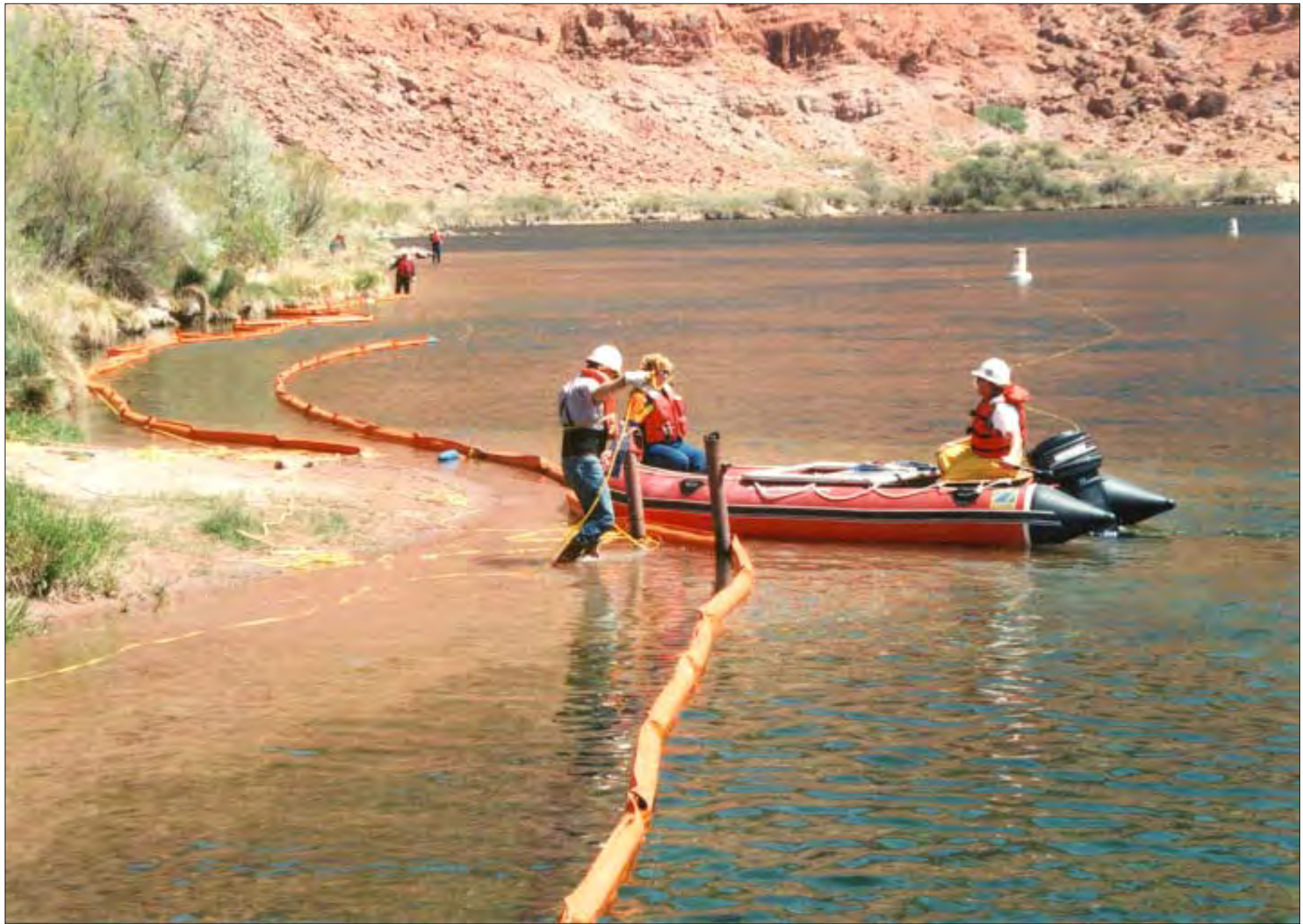
Buoy to Bank Rope Anchor System - Boom Layout on Bank Colorado River - Page, Arizona Area
