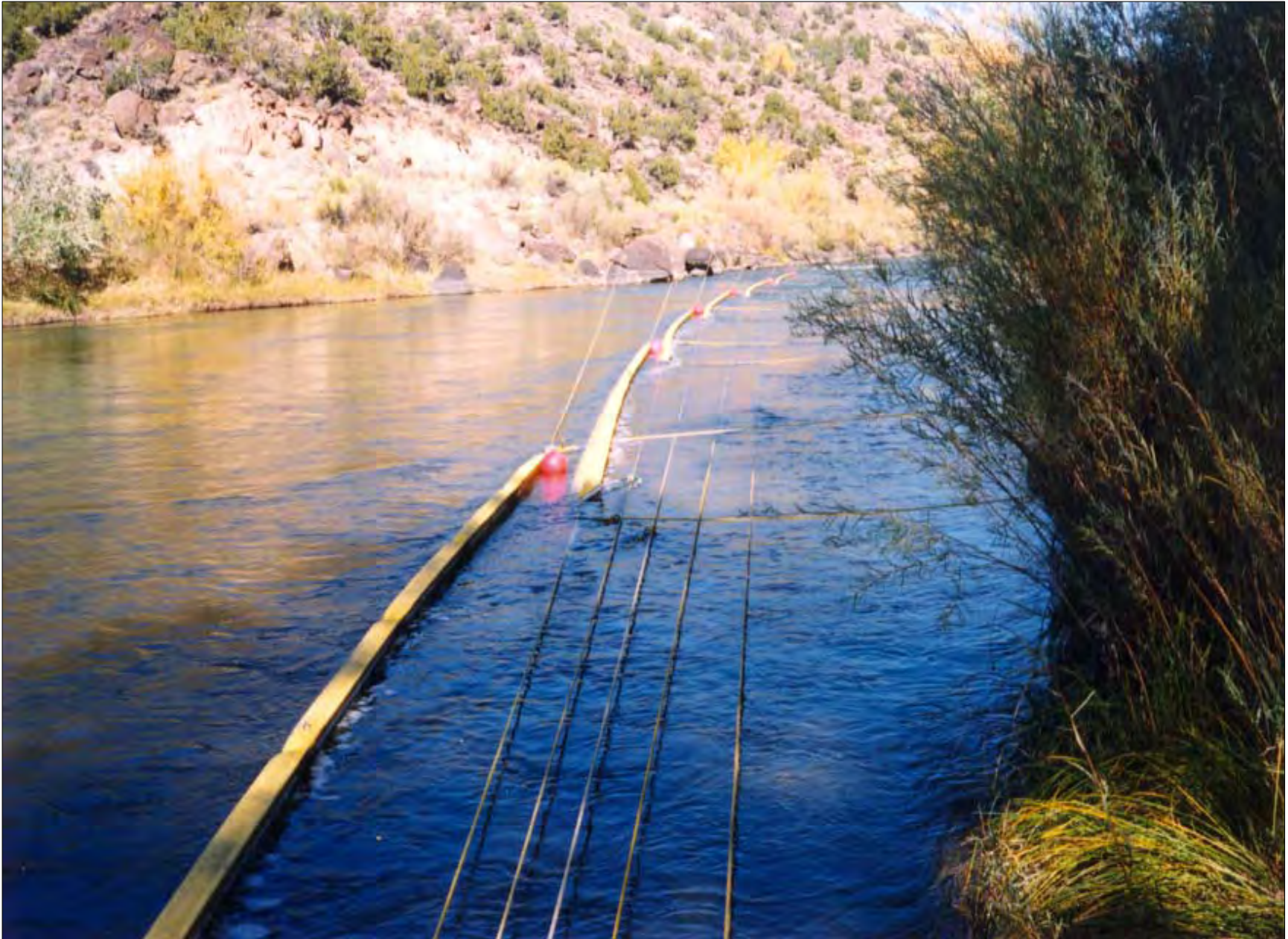
Bank to Bank Rope Anchor System Rio Grande - Taos, New Mexico
