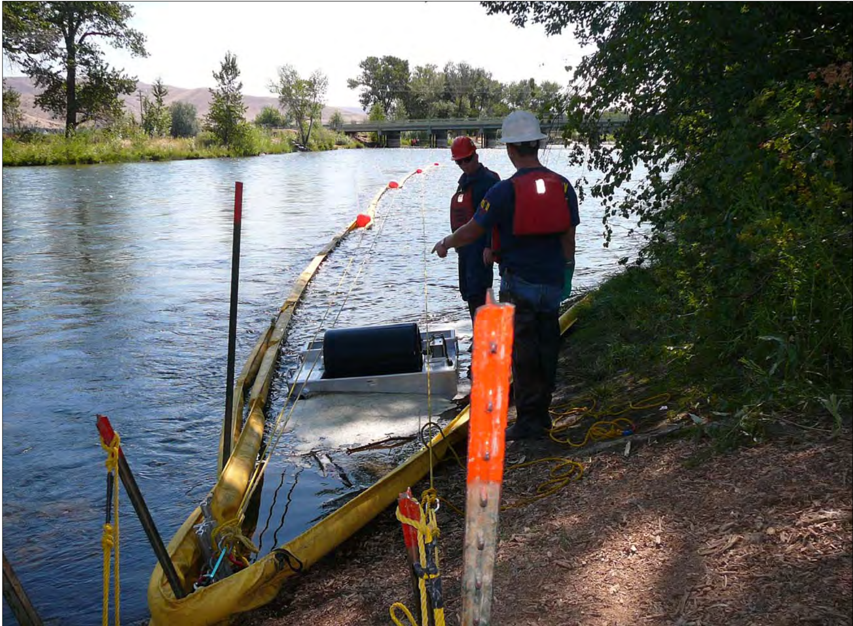
Bank to Bank Rope Anchor System Boise River - Boise, Idaho Area
