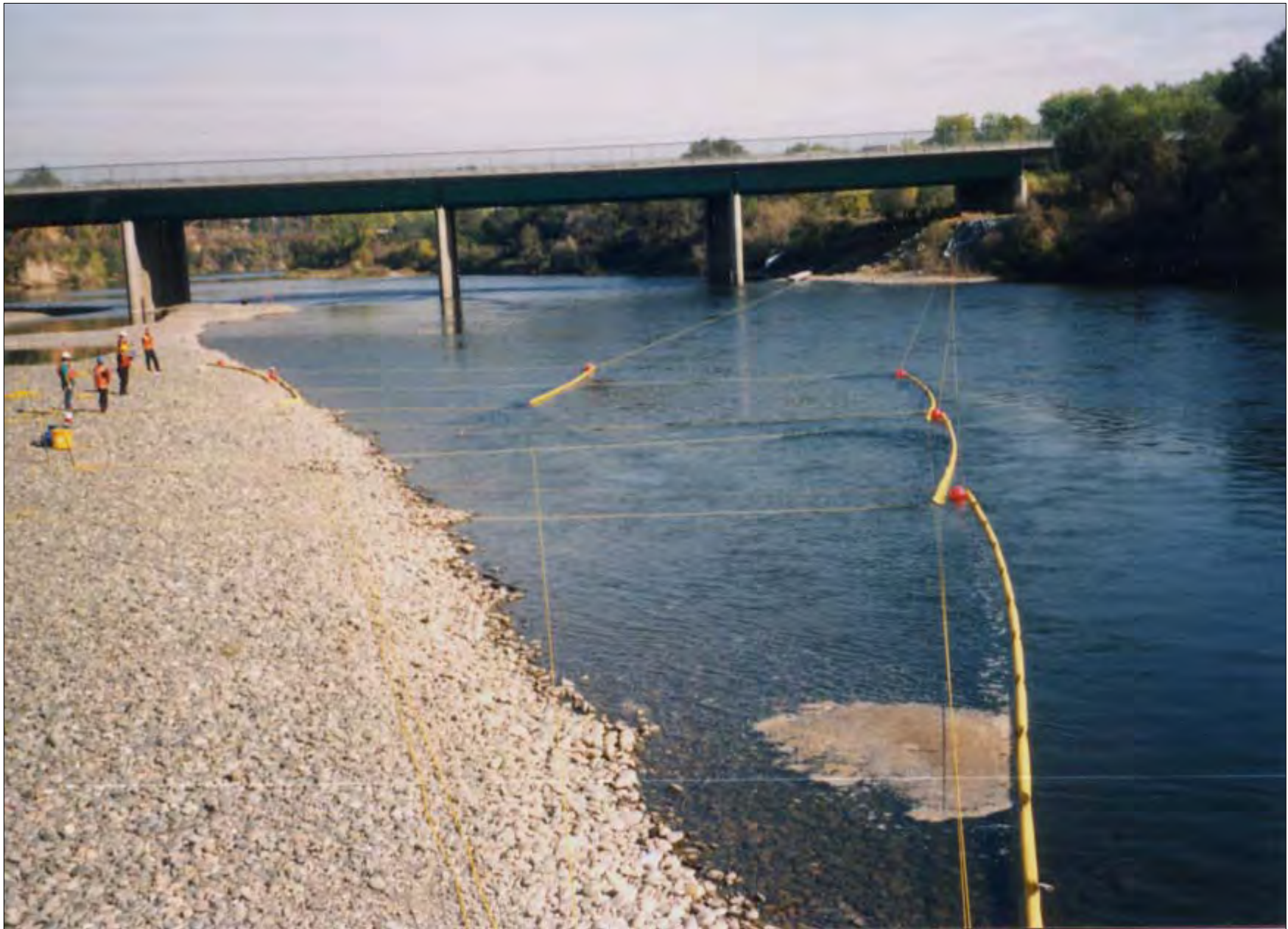
No. 4 - Boom Being Deployed - Bank to Bank Rope Anchor System American River - Sacramento, California
