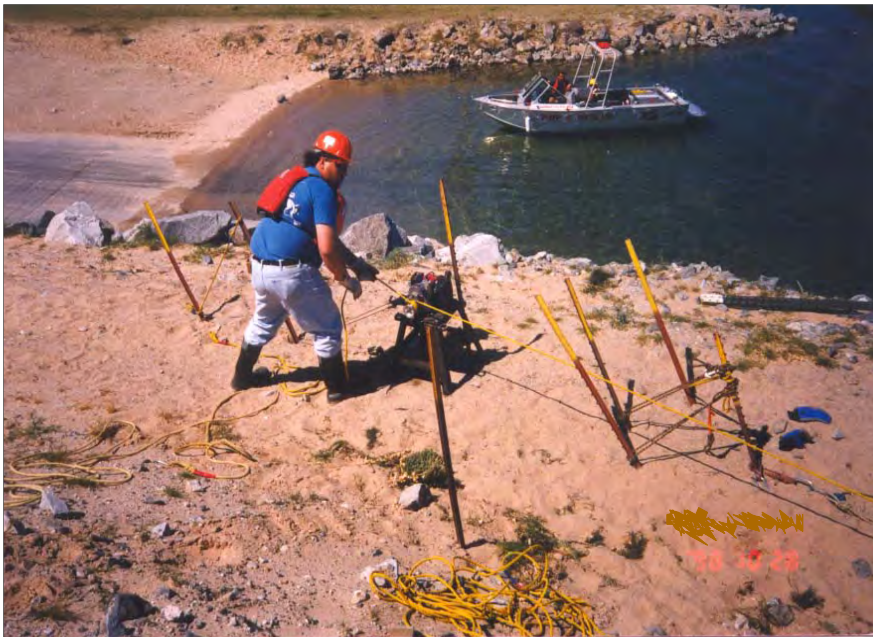
Rope Being Pulled by Power Winch with Side Capstan Mounted on Stand Colorado River - Bullhead City, Arizona Area
