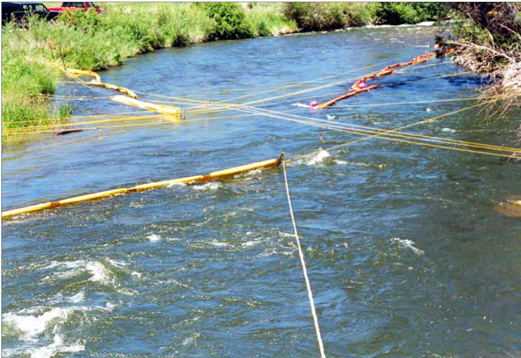
Bridge to Bank Rope Anchor System Open Chevron Cascade Boom Deployment with Deflection Weber River - Coalville, Utah Area
