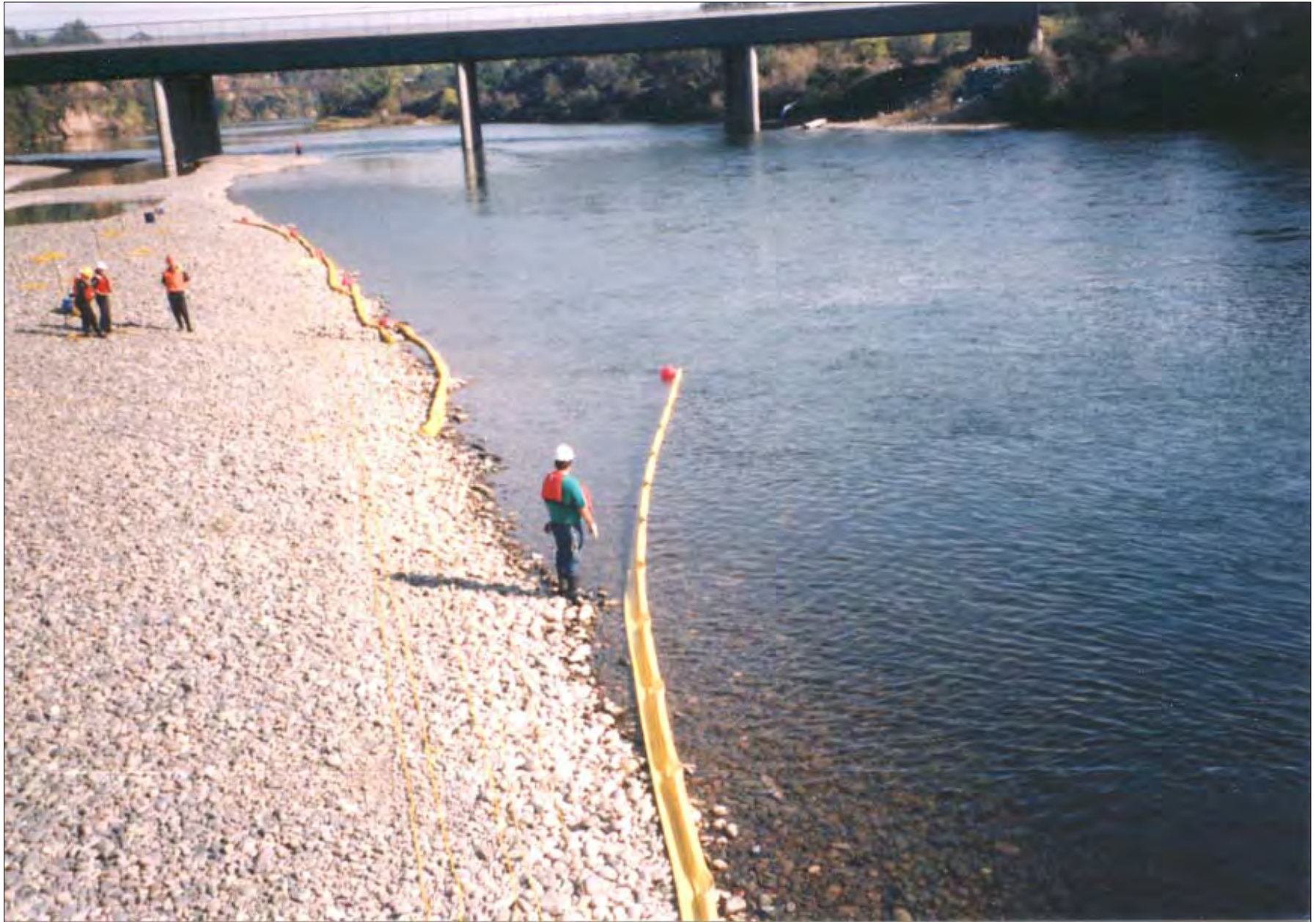
No. 1 - Boom Being Deployed - Bank to Bank Rope Anchor System American River - Sacramento, California
