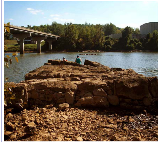
FIGURE 4-12: EXPOSED BRIDGE PILINGS
