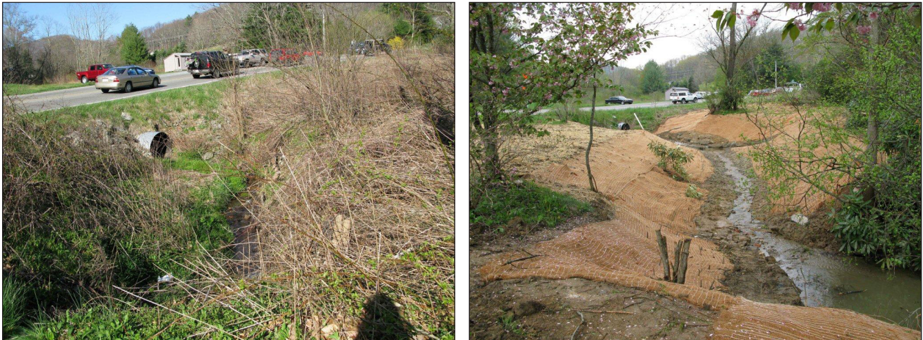
FIGURE 2-23: STREAM RESTORATION EFFORTS ALONG EAST FORK (LEFT: BEFORE; RIGHT: AFTER)
