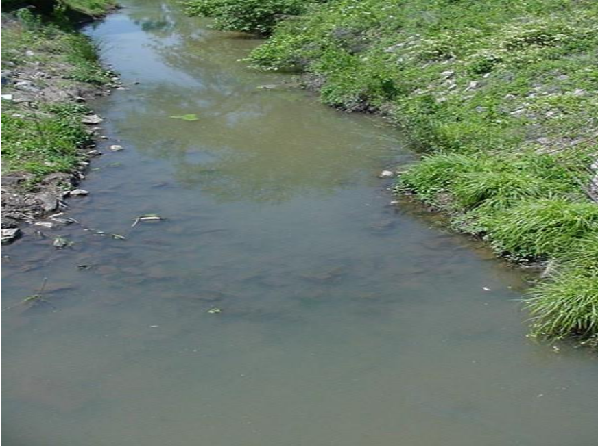
Drain from Greshams Lake (upstream view)
