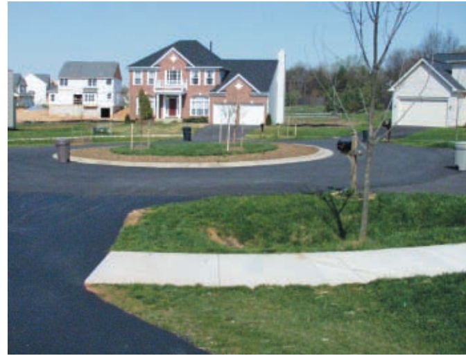
Grassed swales in subdivisions reduce the amount of stormwater pollution entering rivers and streams.
