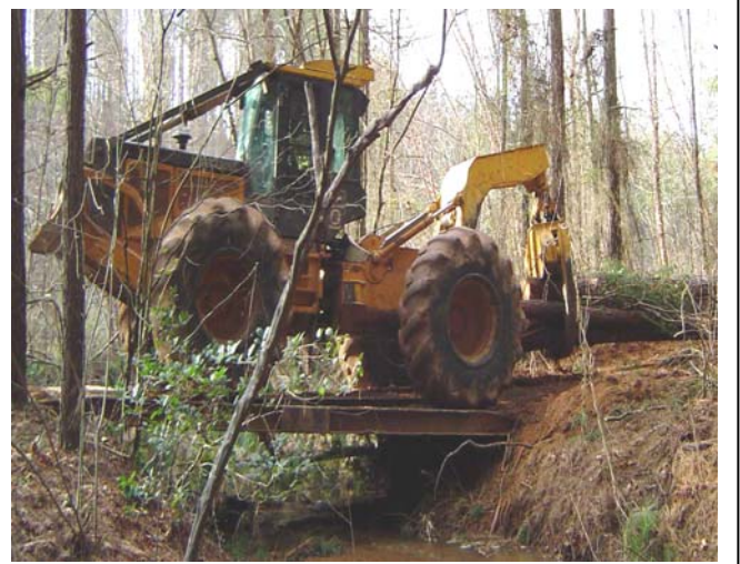
Figure 7-1 Portable Bridgemats Protecting a Stream Crossing
