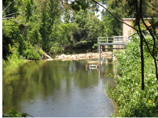
Hendersonville Water Intake Structure
