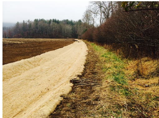
Grassed waterway installation
