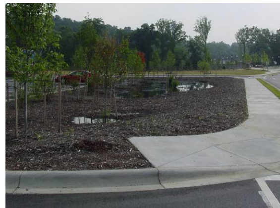
Following a rain event, stormwater enters the bio-retention area where it is absorbed by mulch and soil and is taken up by plants.
