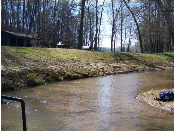
Lack of woody vegetation in the riparian area.
