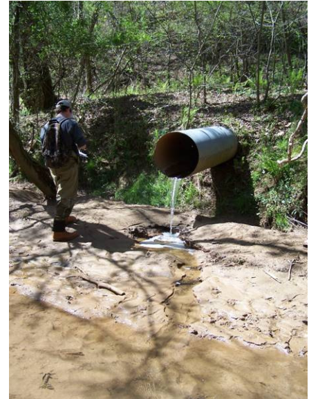
Pipe outfall entering Hunting Creek.
