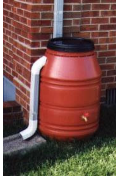
A rain barrel is attached to a downspout and collects rain water.
