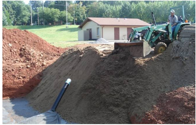
The depression is filled with a soil medium that allows water to slowly infiltrate into the ground while removing pollutants through filtration.
