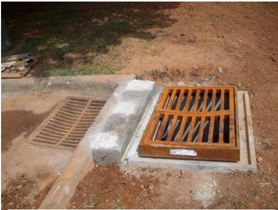
Water from the parking lot flows into a storm grate....
