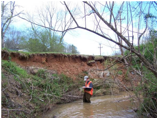
Eroding stream bank along Hunting Creek lacking woody riparian vegetation.
