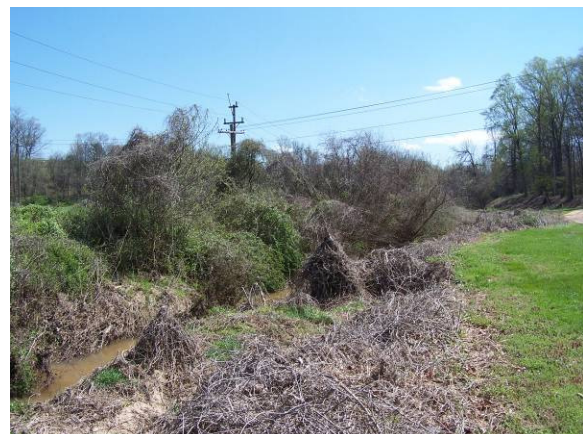
Power lines crossing Hunting Creek overhead.
