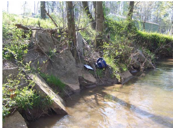
Bank armoring with large concrete slabs along Hunting Creek.
