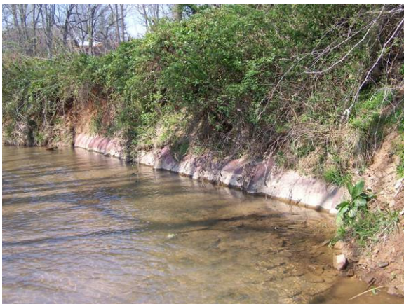
Pipe utility parallel to Hunting Creek along stream bottom.
