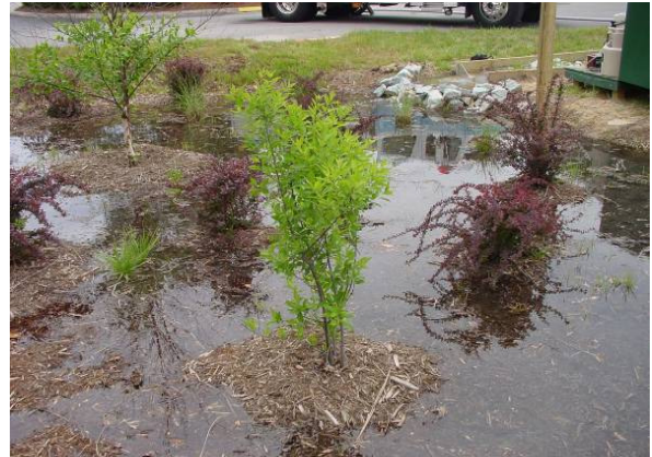
A bio-retention area effectively captures runoff, preventing large volumes of polluted runoff from entering a stream.
