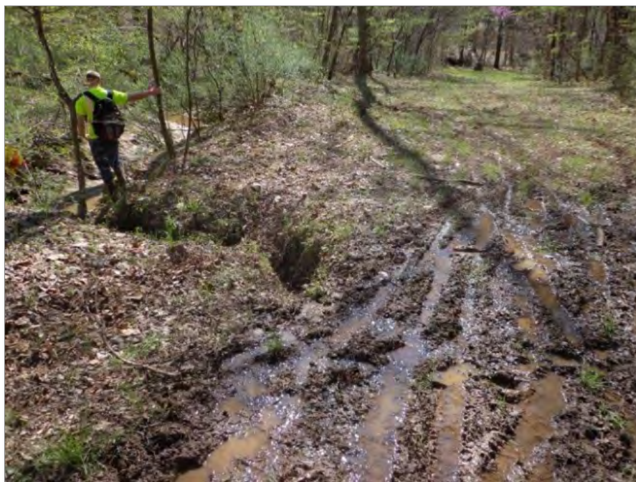
Photo 5. Drainage channel with headcut progressing across utility easement
