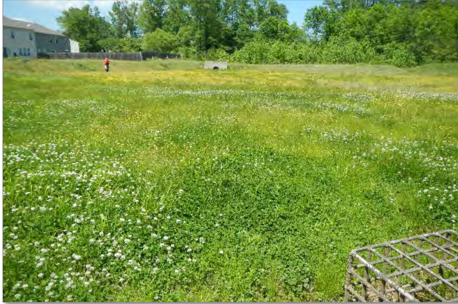
Photo 18. SCM 00236 – Example of dry pond that could be converted to a stormwater wetland with a simple structural retrofit
