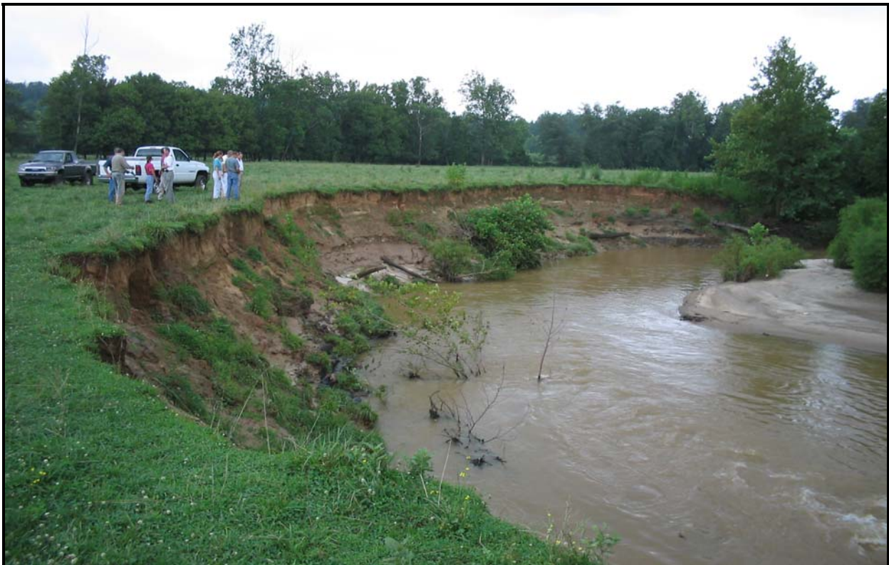
Figure 7: Streambank erosion along Lower Creek, 07/31/03 (LL07)
