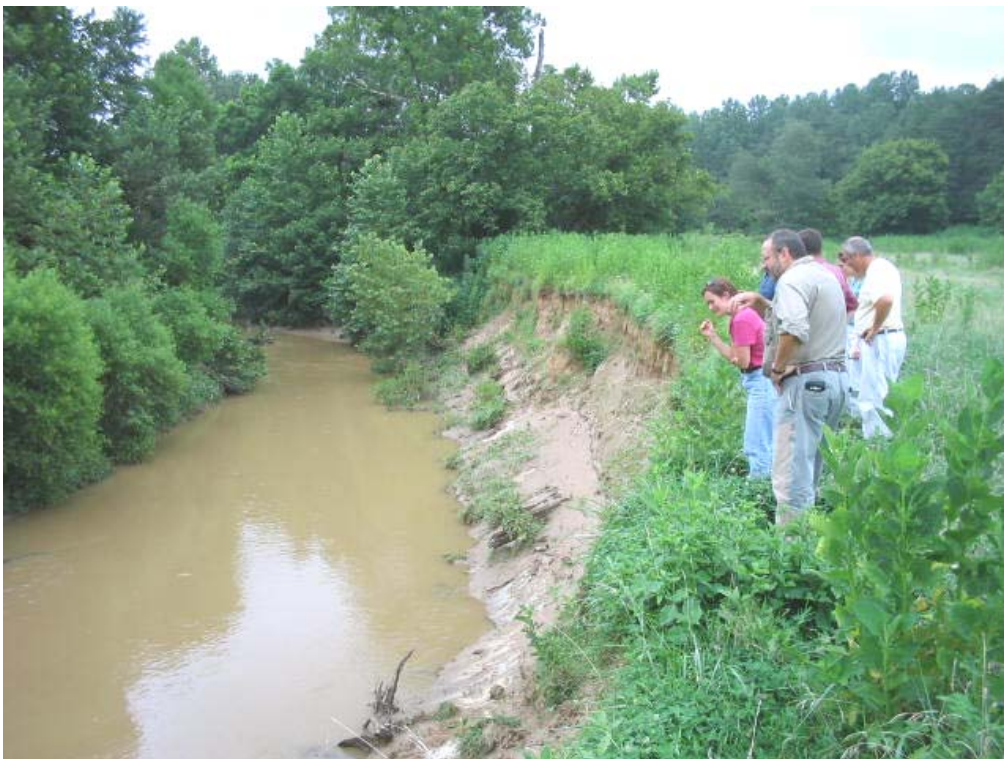
Figure 18: Lower Creek (potential NCWRP project site), facing upstream
