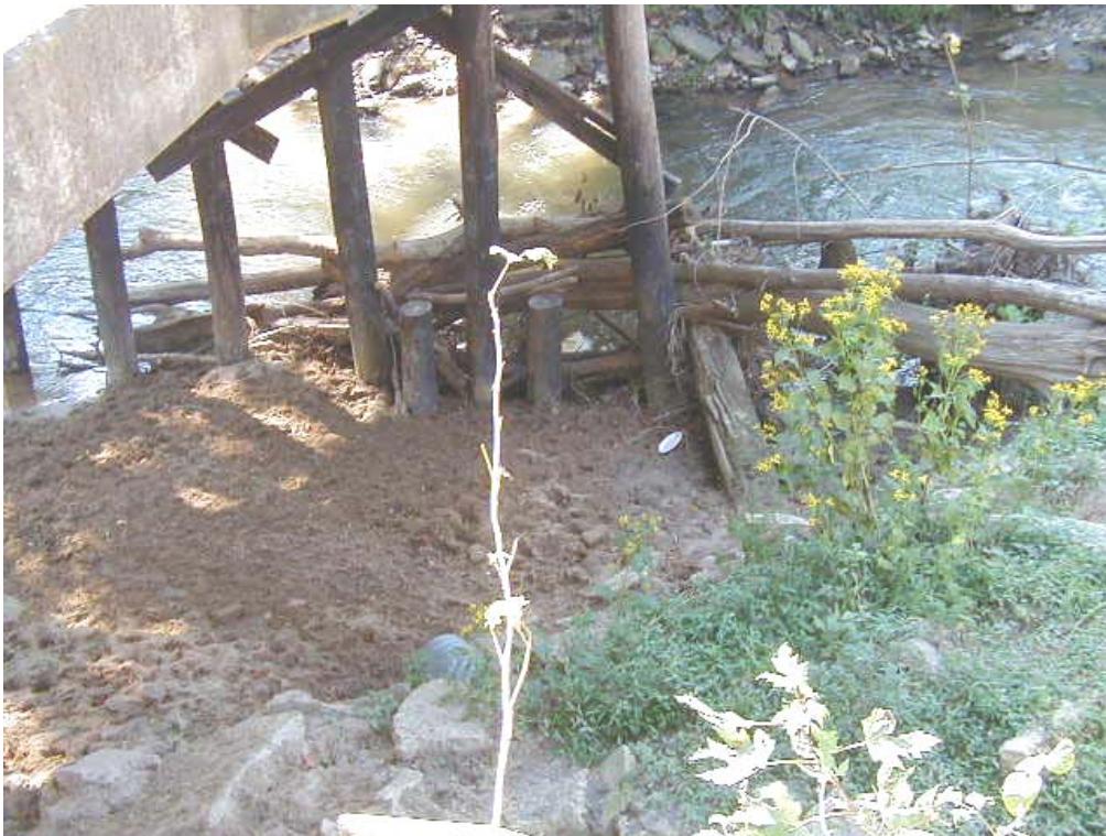
Figure 14: Lower Creek at Rocky Road bridge, facing upstream
