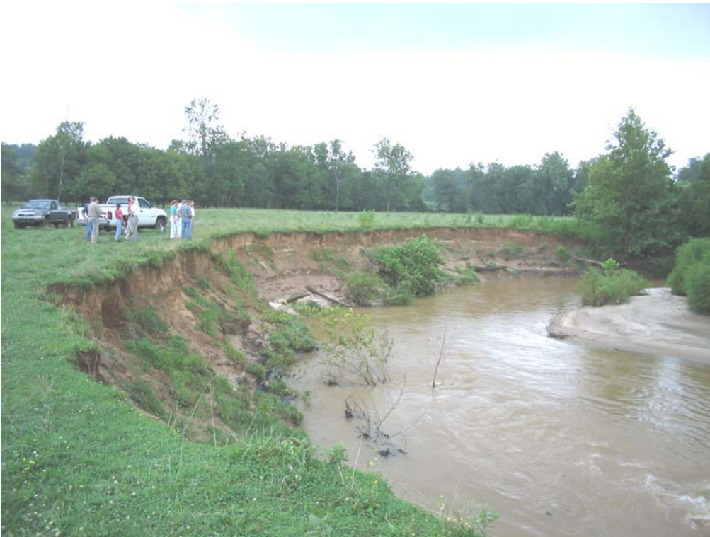
Figure 16: Lower Creek (potential NCWRP project site), facing downstream
