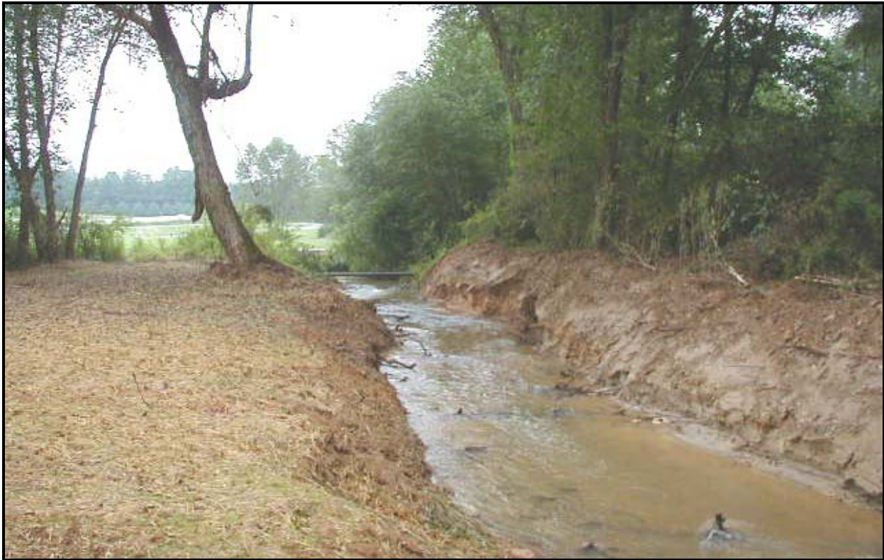
Figure 8: Construction activities along Zacks Fork at soccer complex, 09/04/03 (UL07)
