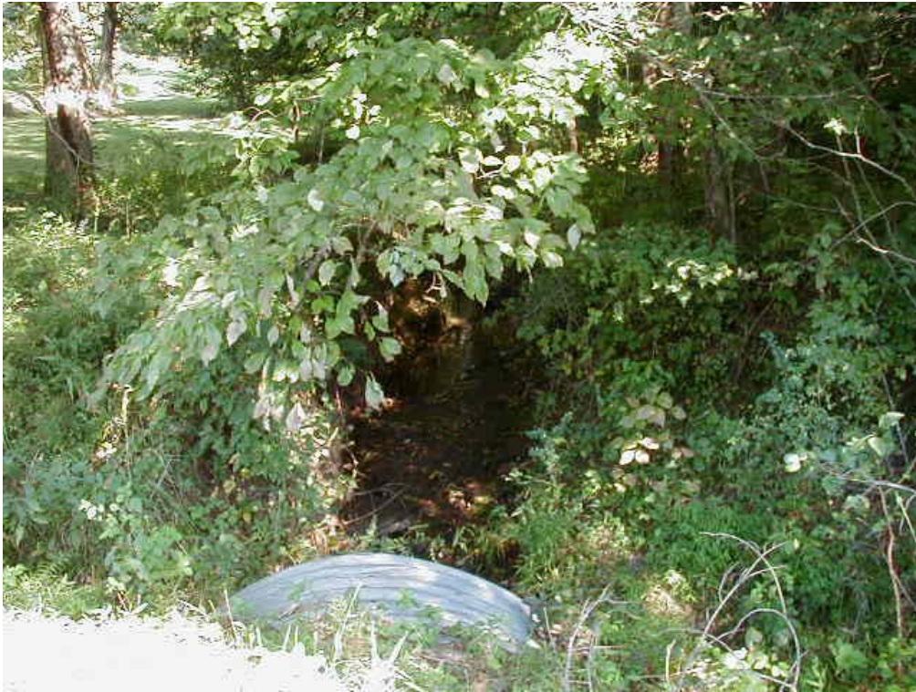
Figure 56: Unnamed tributary to Lower Creek at Craigs Mountain Road, facing upstream
