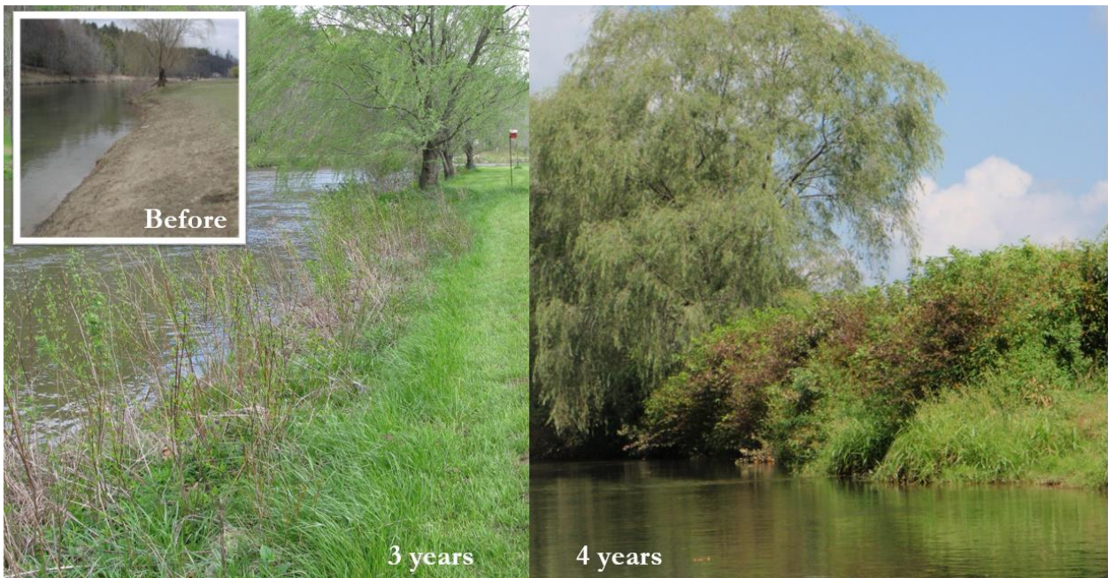
Streambank stabilization accomplished with a native riparian buffer.
