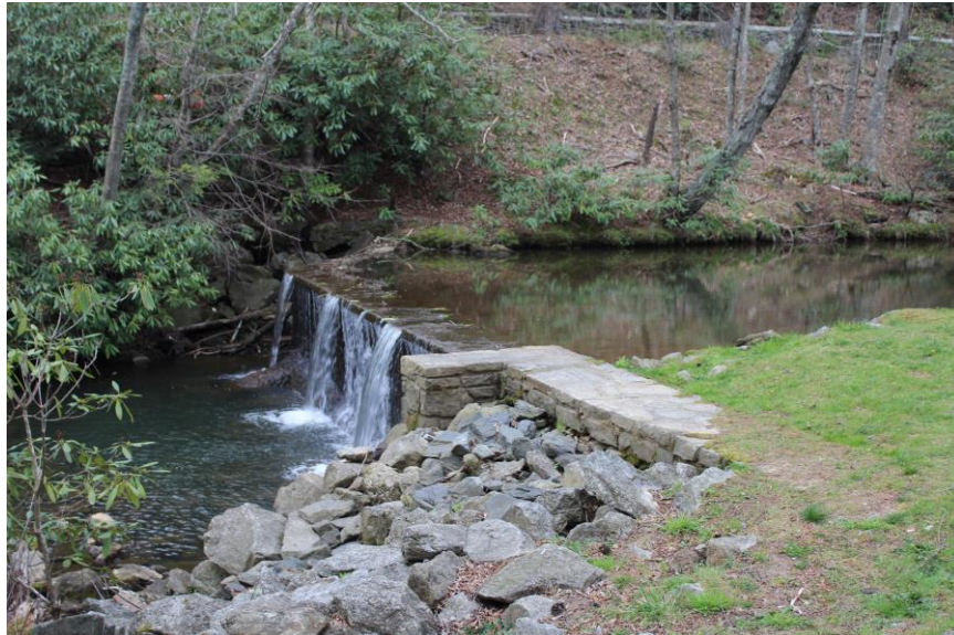
Dam at the at the inflow of the Middle Fork into Chetola Lake
