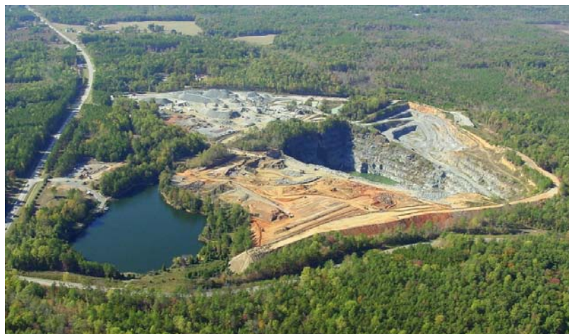
Existing reservoir is on the left. Active quarry pit is advancing from the right.
