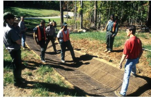
Figure 9. Turf reinforcement mats increase allowable velocities for grassy swales, making swale use more possible.
