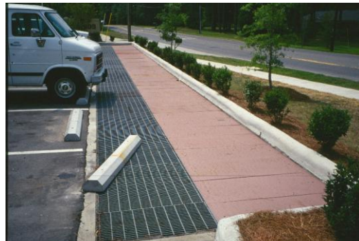
Figure 7. Sand filters can be designed to sustain vehicular traffic or not as is the case at this site in Durham.
