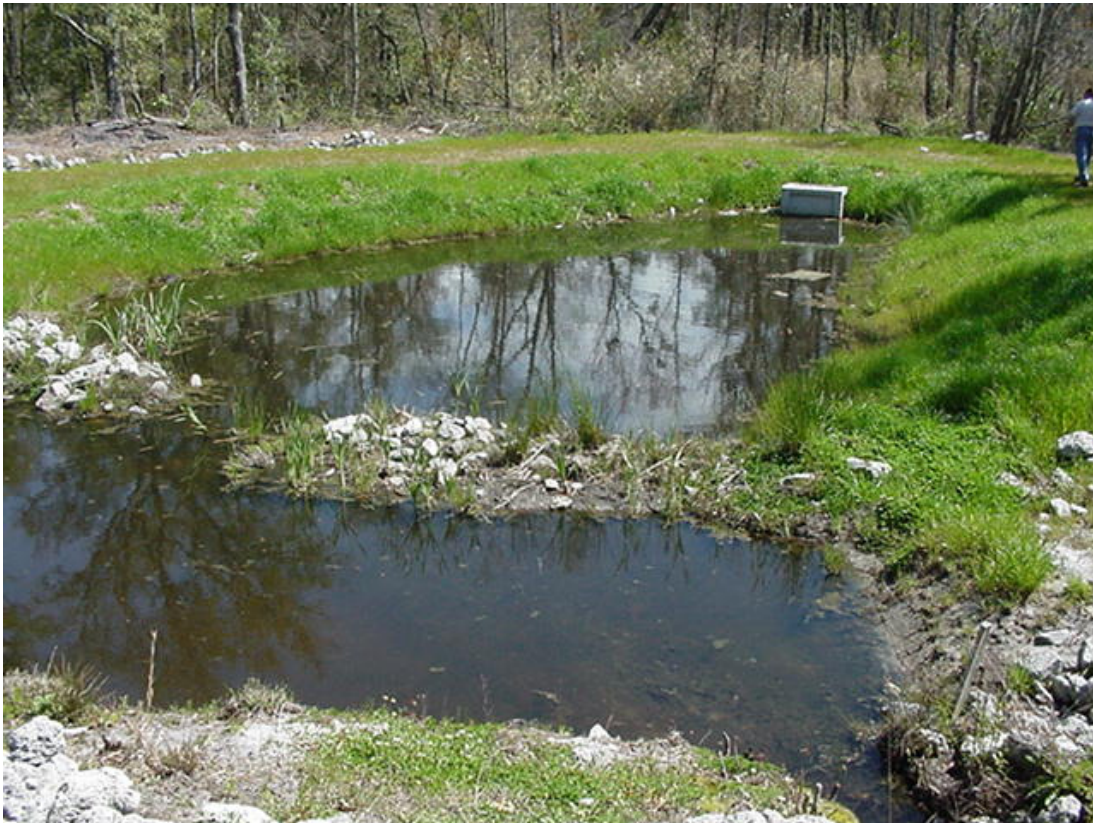
Figure 10-1 Permanent Pool of Water in Wet Detention Basin
