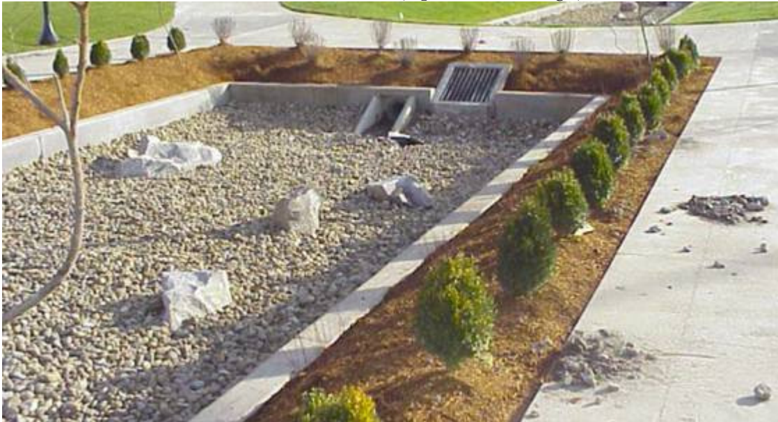
Figure 11-1a Surface Sand Filter (Open Basin Design)
