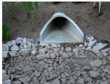
Figure 12-2b Bioretention Cell with Pretreatment: Forebay
