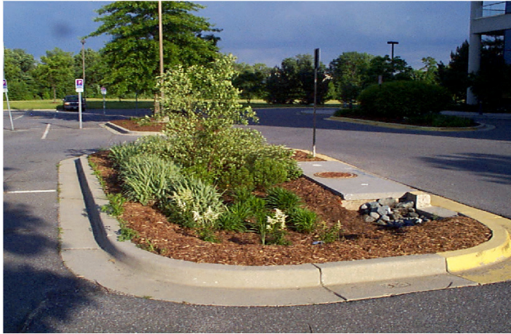
Figure 12-1 Bioretention in Parking Lot Island
