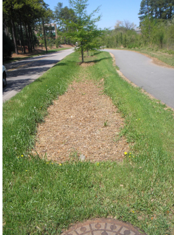
Figure 12-2a Bioretention Cell with Pretreatment: Gravel and Grass (Needs Maintenance)
