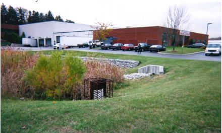
**Figure 17-1**Dry Extended Detention Basin with Shallow Marsh
