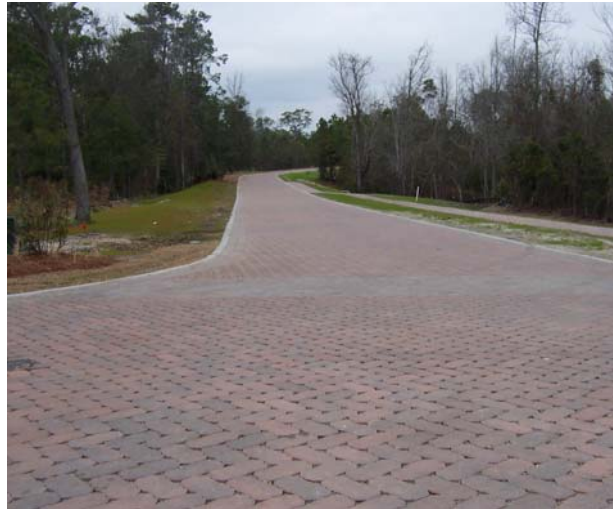
Figure 18-12b. Perimeter edge restraint used with PICP
