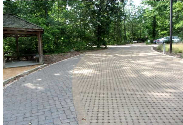
Figure 18-1. Permeable pavement reduces runoff volumes and pollutants.
