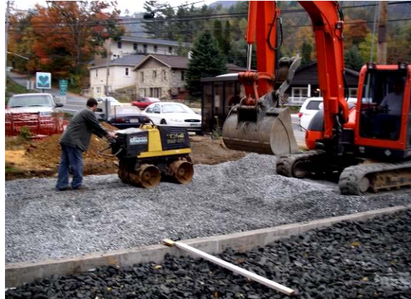
Figure 18-20. Compacting the open-graded aggregate base Source: NCSU-BAE
