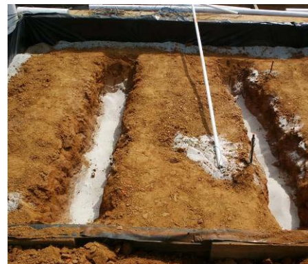
Figure 18-17. Trenching used to increase the soil infiltration rate. Source: Tyner
