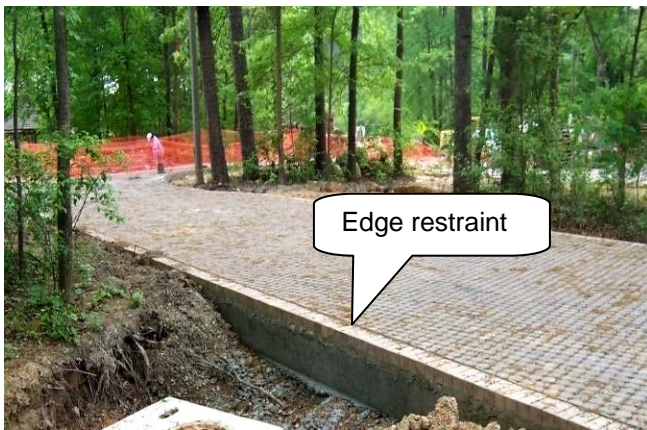
Figure 8-11. Edge restraints for the pavers, typically concrete curbs are required for PICP.
