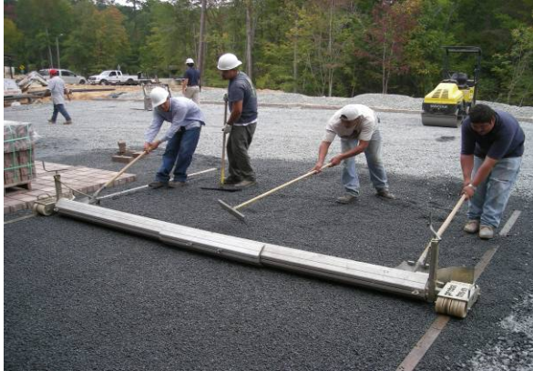
Figure 18-21. A 2 in. thick bedding course of aggregate is being screed smooth prior to placing the concrete pavers.
