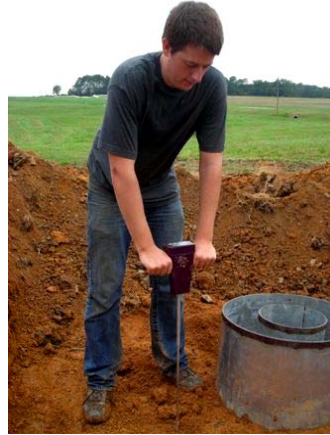
Figure 18-6b. Soil boring tests are required for permeable pavements. Source: NCSU-BAE
