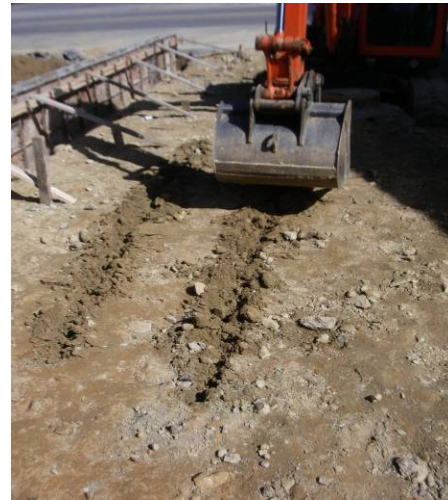
Figure 18-16. Ripping the soil subgrade increases its infiltration rate. Source: Tyner
