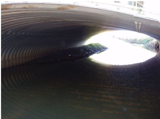
Downstream through structure
