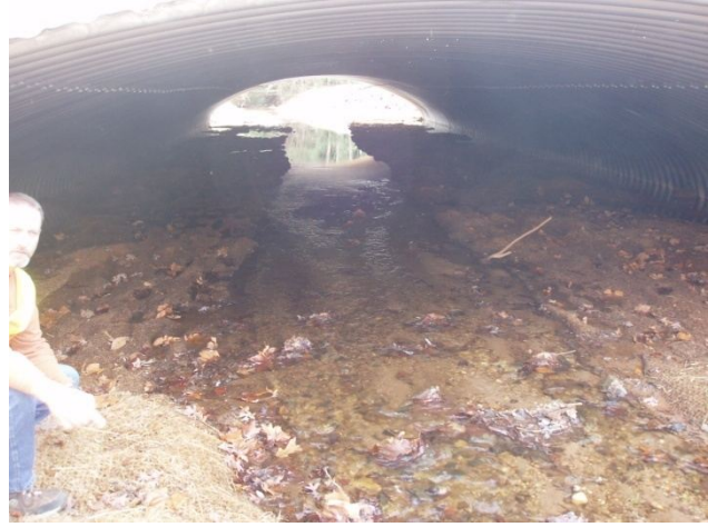
Downstream through structure
