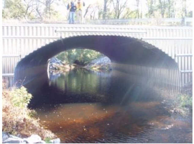
Inlet of structure
