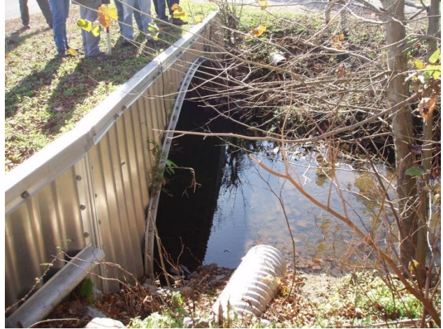
Outlet of structure
