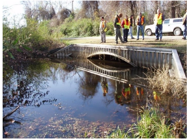
Inlet of structure
