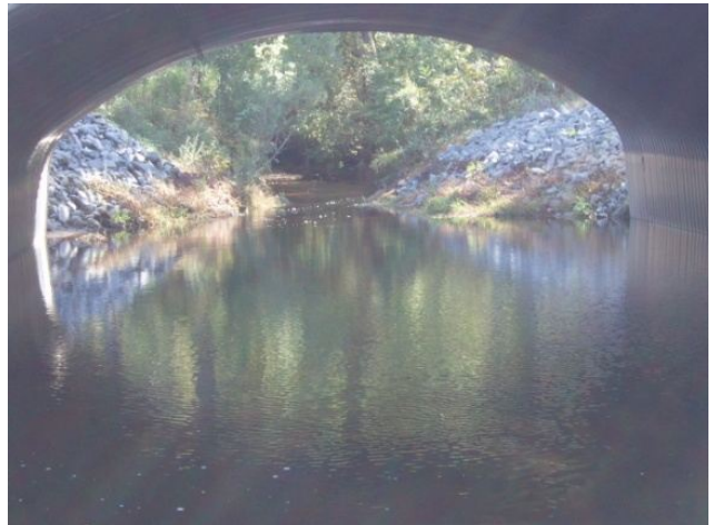
Upstream through structure
