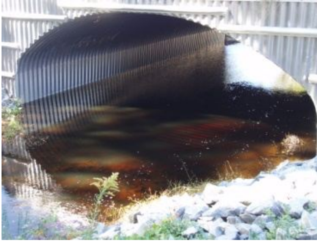
Outlet of structure
