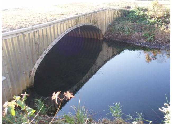
Outlet of structure
