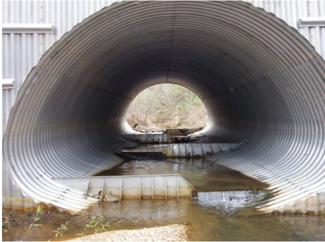
Upstream through structure
