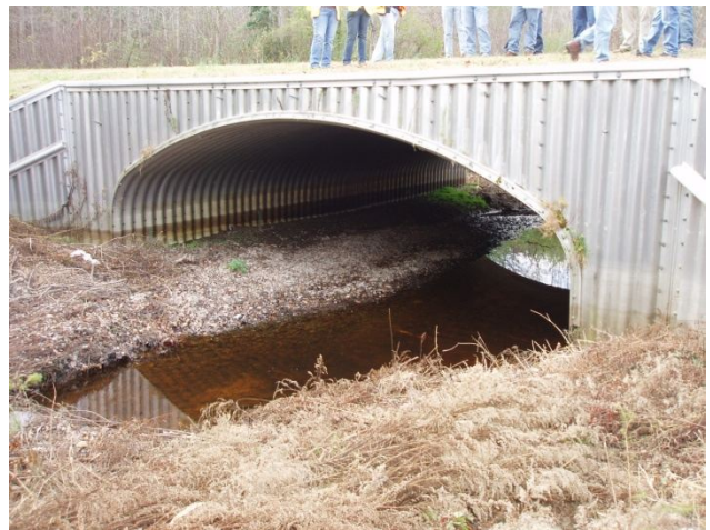
Downstream side of structure
