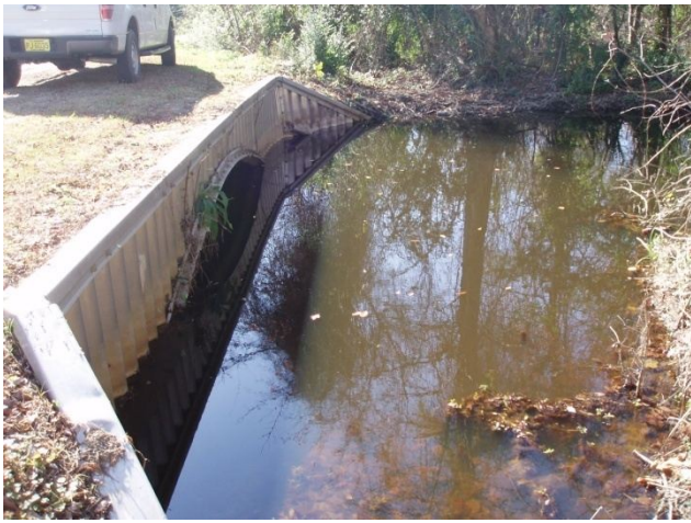
Outlet of structure
