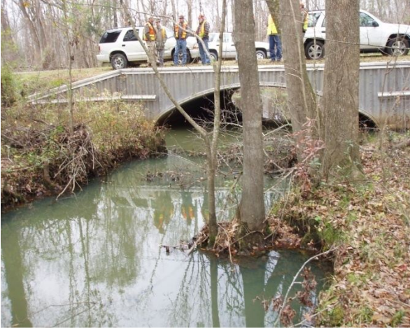
Outlet of structure
