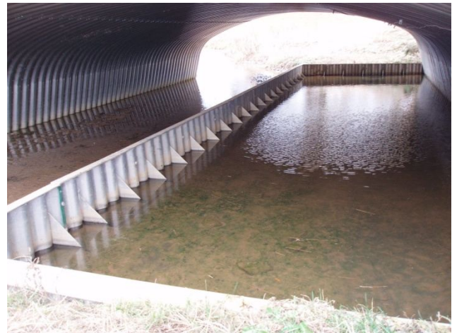
Downstream through structure (knee wall on right)
