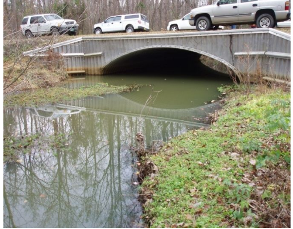
Inlet of structure
