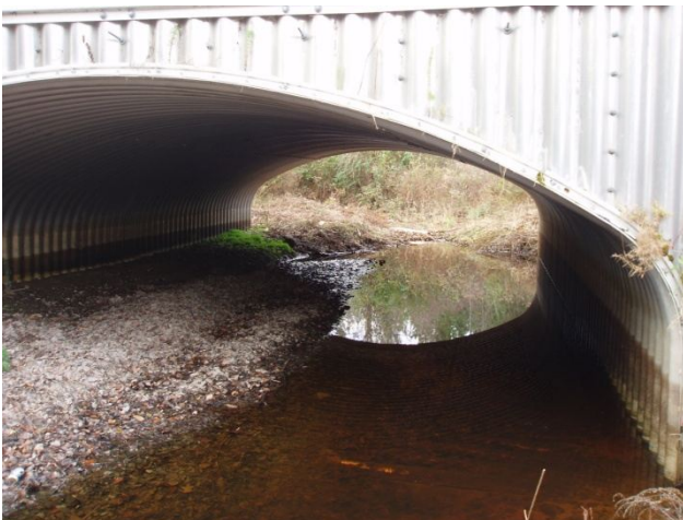
Upstream through structure
