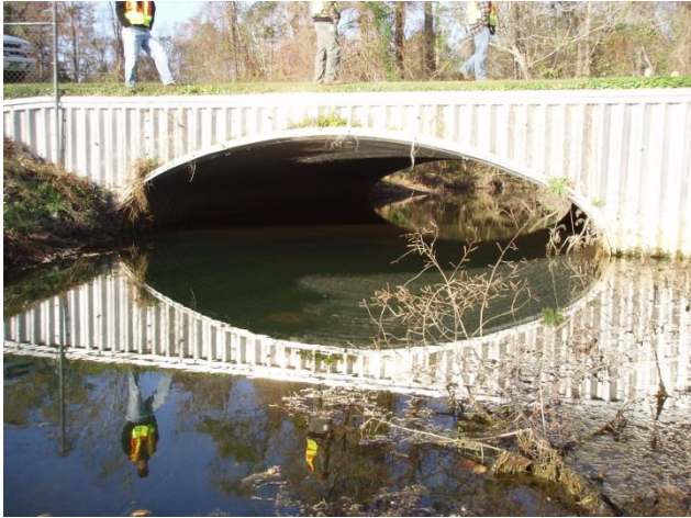
Inlet of structure
