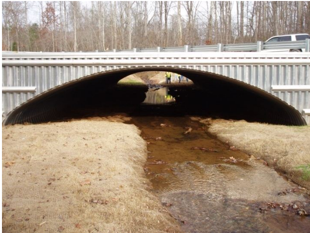
Downstream at structure
