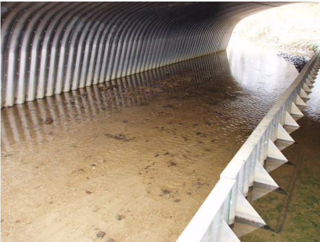
Downstream through structure
