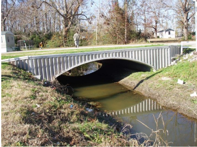
Outlet of structure
