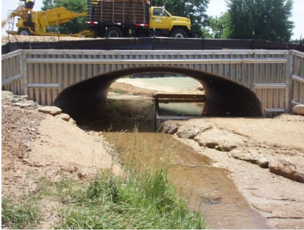
Inlet of structure (under construction)
