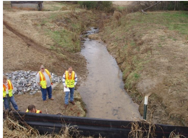
Upstream of structure
