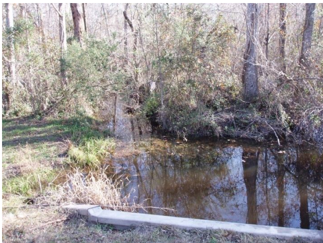
Upstream of structure
