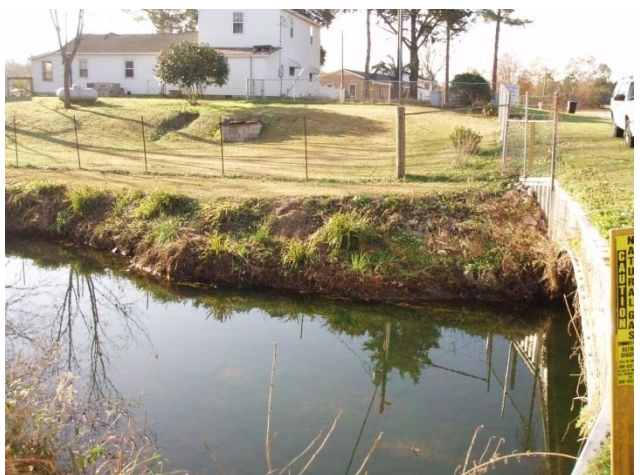
Upstream of structure
