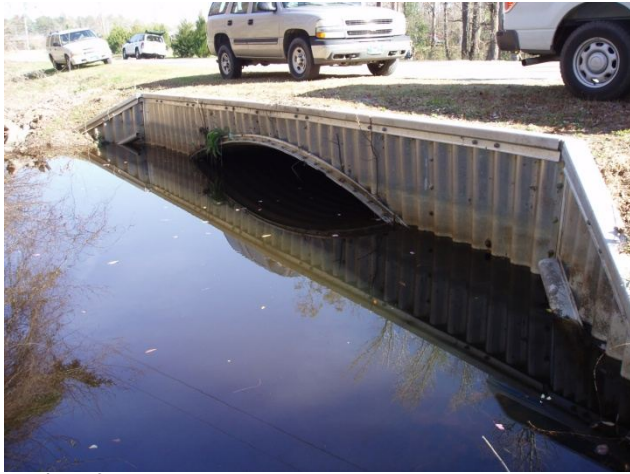
Inlet of structure
