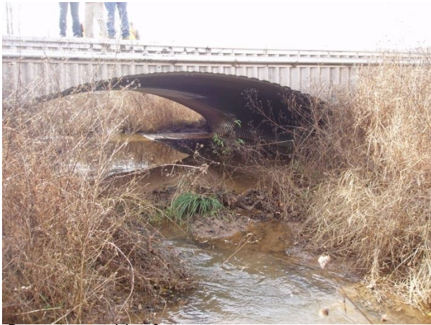
Downstream side of structure
