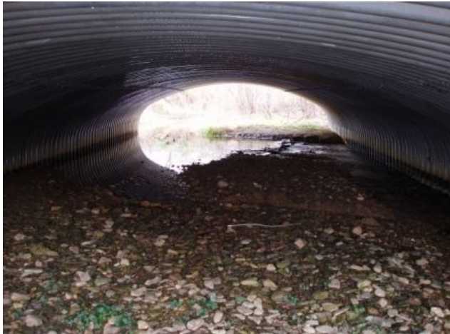
Upstream through structure
