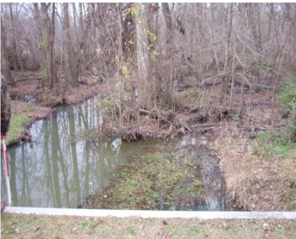
Upstream of structure
