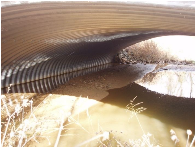
Downstream through structure
