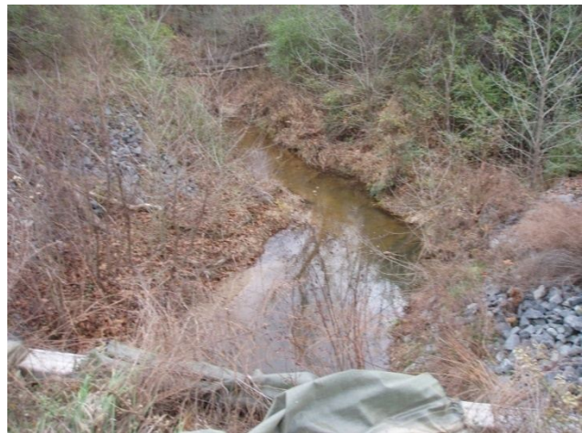
Upstream of structure
