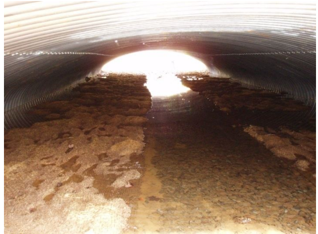
Upstream through structure
