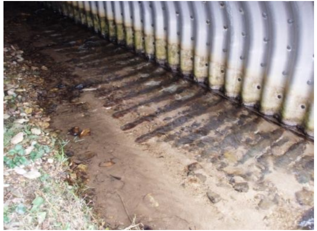
Main flow at outlet of structure
