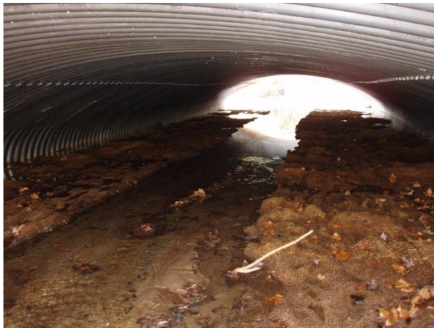
Downstream through structure
