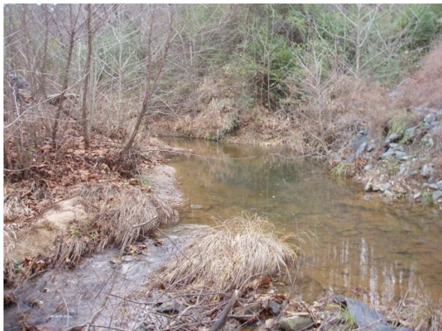
Upstream of structure
