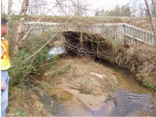
Outlet of structure
