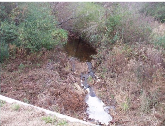
Upstream of structure
