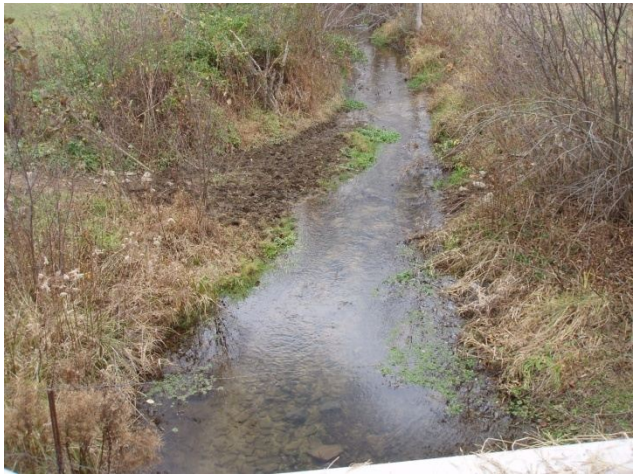
Upstream of structure (horse crossing on left side middle)
