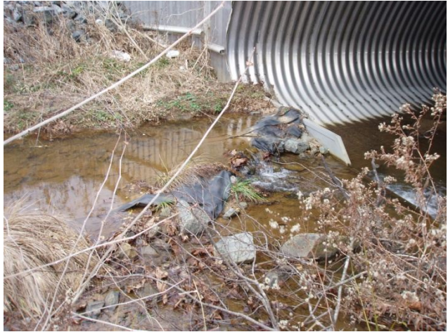
Intlet of structure
