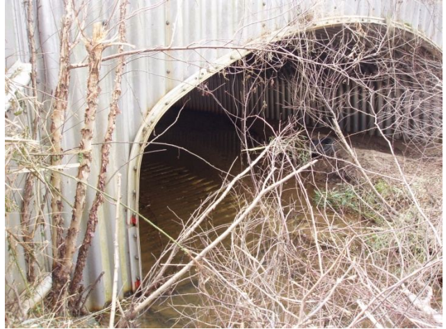
Inlet of structure
