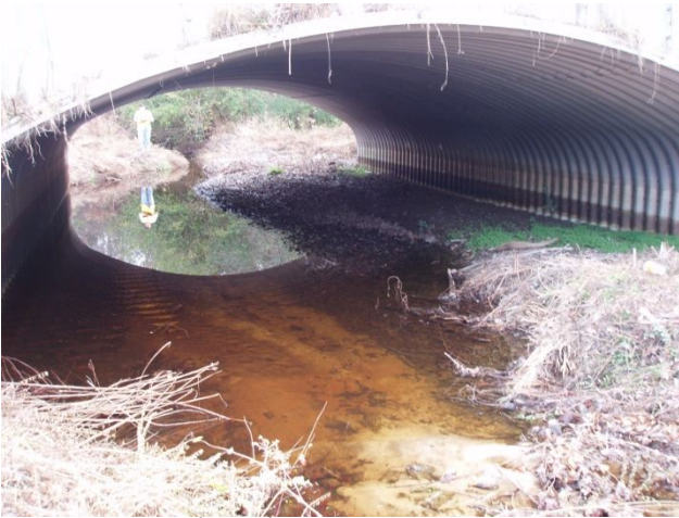
Downstream through structure
