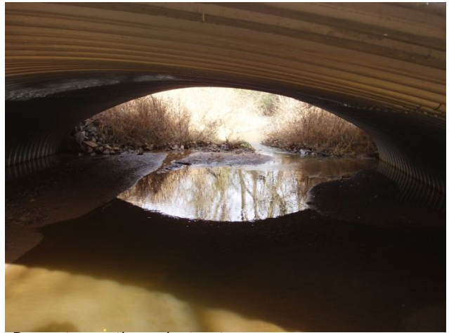
Downstream through structure
