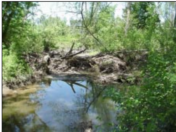
Debris dam across Swift Creek above the crossing at SR 1152, Wake County.
