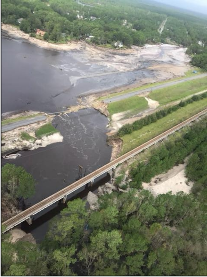
Figure 4. Aerial view of the Boiling Springs Lake Breach) Caused by Hurricane Florence flooding, September 17, 2018. (Brunswick County Sheriff's Department)
