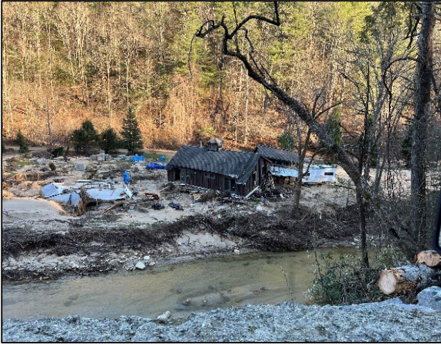
Home swept off foundation, Hungry River downstream of SR 1799.
