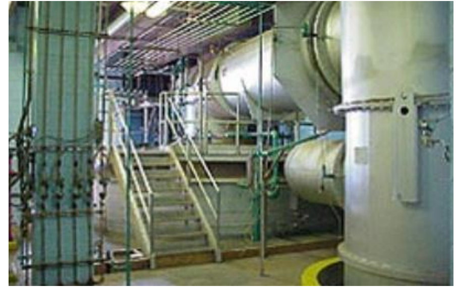
Greensboro Incinerator, Source
