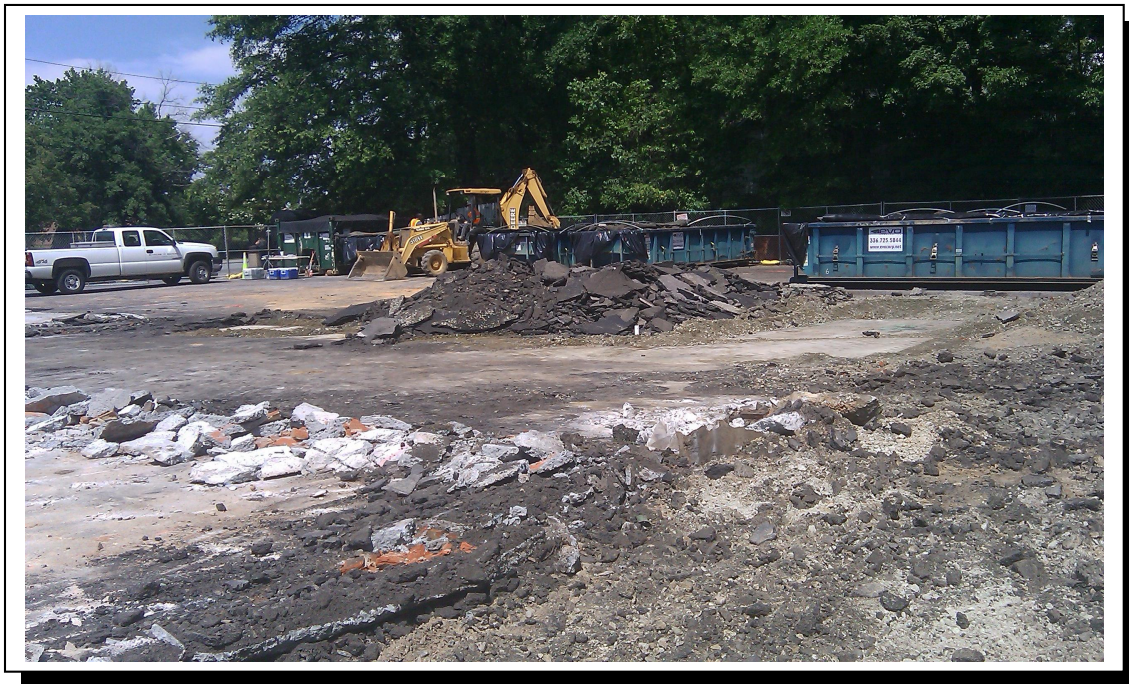
Description: View of removed asphalt to fill roll-off container #13123684.
