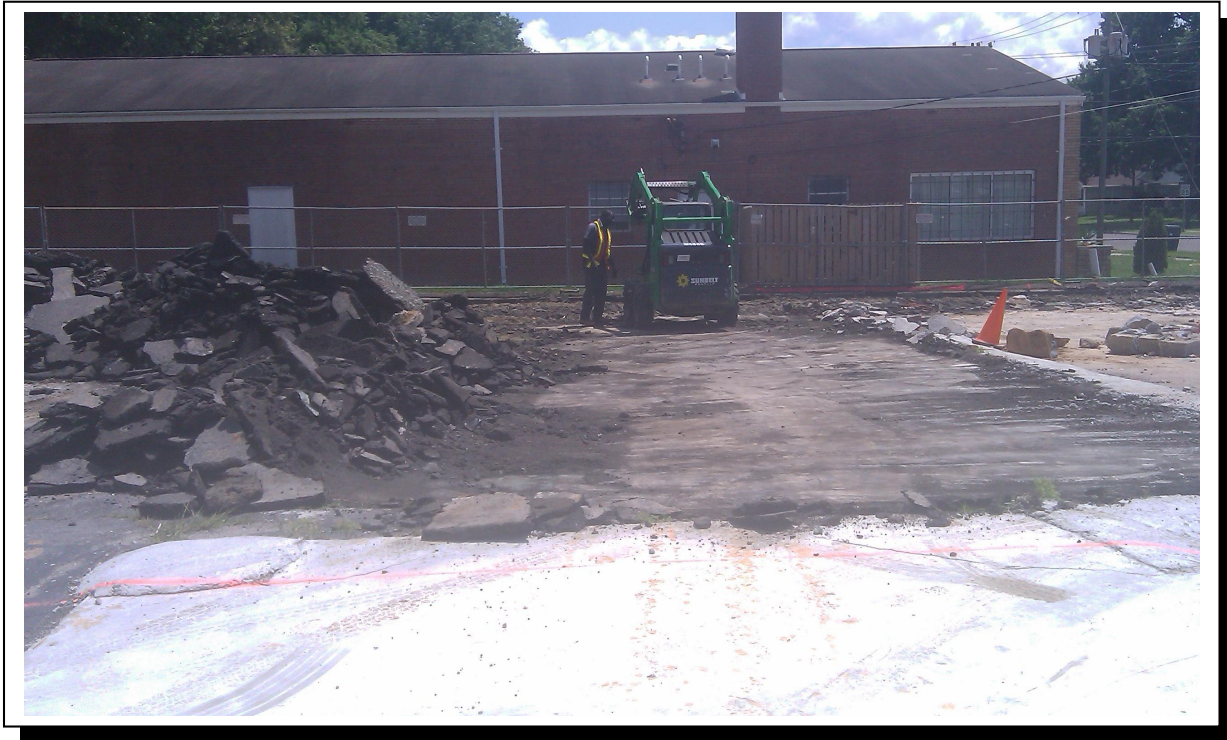
Description: View of removed asphalt to fill roll-off container #13123683.
