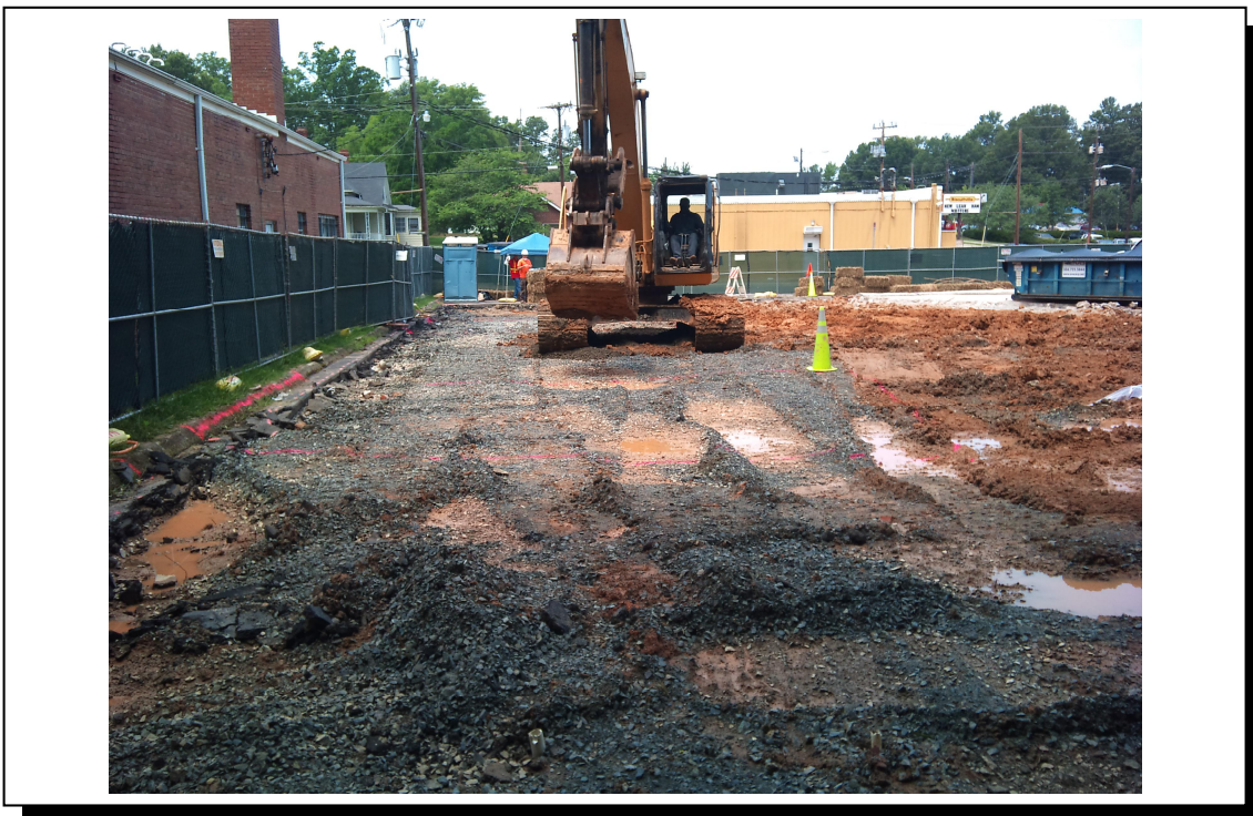
Description: View of secondary source area prior to excavation.
