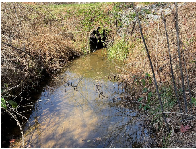
PP-37: Reach UT4A, upstream, Station 10+25
