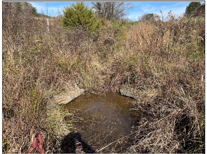
PP-48: Reach UT5, upstream, Station 10+50
