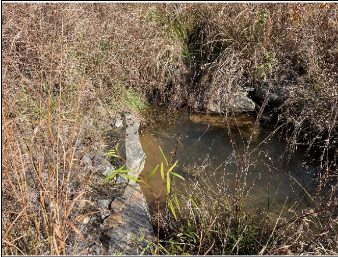
PP-43: Reach UT5, upstream, Station 13+60
