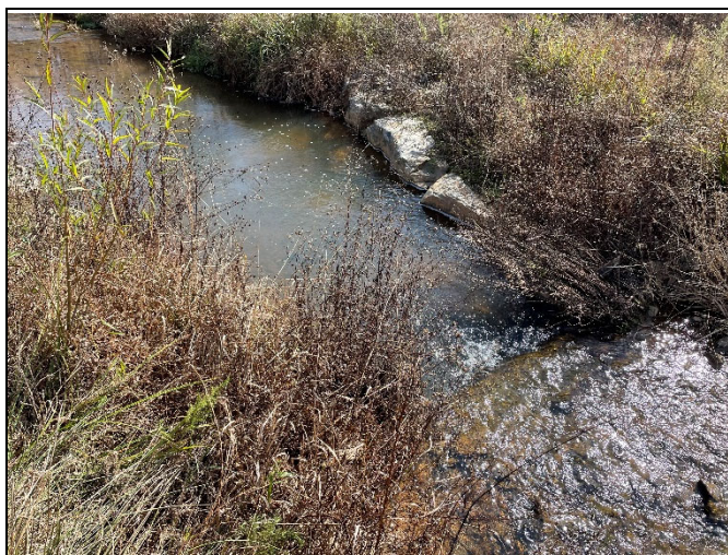
PP-21: Reach 7, downstream, Station 24+00
